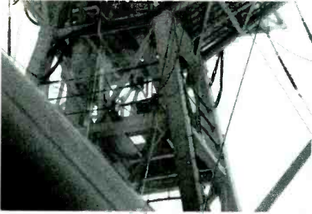
Close up of the main mast showing numerous bonding wires and, if you know where to look, the feedlines for the HF wire antenna.
