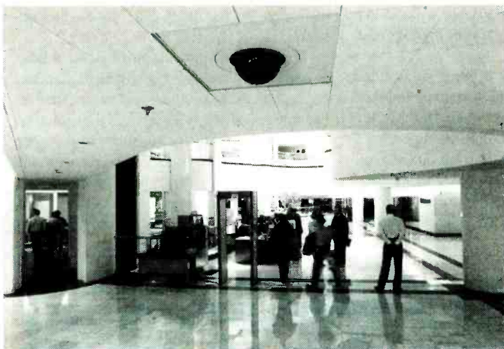
The Sensormatic SpeedDome (top, foreground) provided video surveillance at the main security checkpoint at ACOG headquarters.
