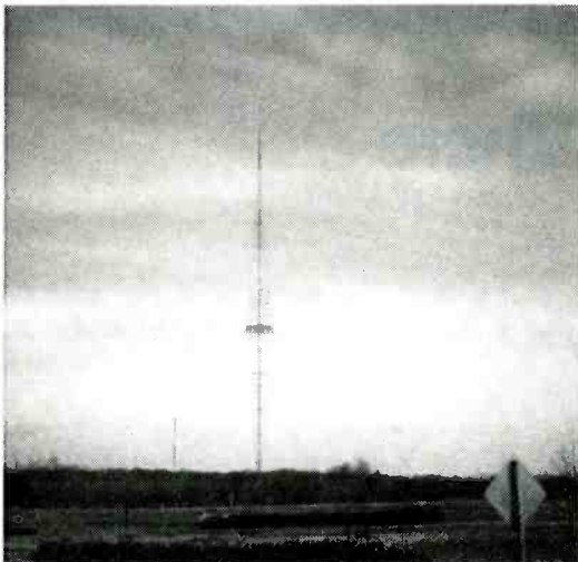
This impressive tower belongs to WSM 650. If you come to Middle Tennessee, you can see it along Interstate 65 in Brentwood. As there's only one tower on the site, you can tell WSM is a non-directional station (see September 1995 American Bandscan).
