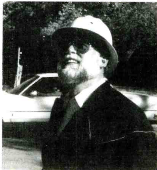
Gene Jameson, division engineer for the Public Service Company of New Mexico, watches as workers in a cherry picker look for loose hardware that could be arcing and causing radio interference.
