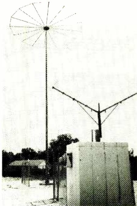
Figure 1. Longwave Beacon "HK" (332 kHz) near Chicago, IL, also includes a V-shaped 75 MHz marker beacon antenna.
