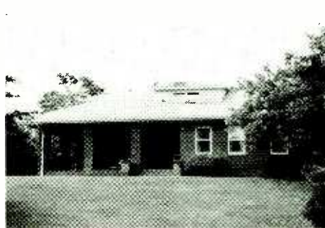
RCA built housing on the Ryder's Cove property for their employees. These homes were occupied by WCC personnel until the station was shut down.
