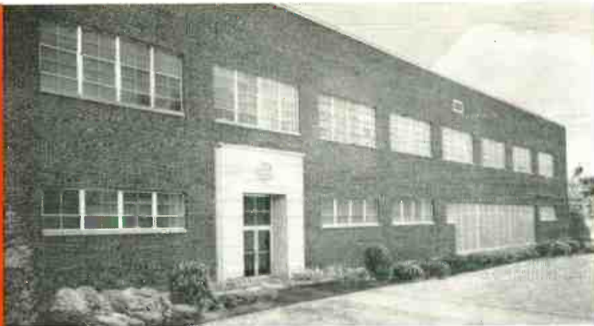
Silicon production facilities of the Electronic Chemicals Division of Merck & Co., Inc. in Danville, Pennsylvania.
