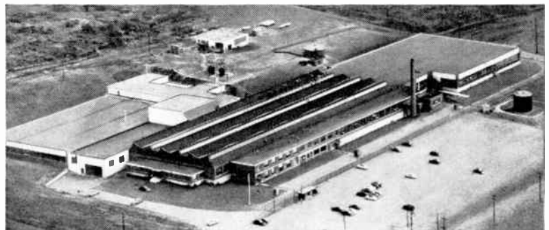
G-E POWER TUBE PLANT AT SCRANTON, PA. High-volume tubes such as thyratrons and parallel-plane tubes are precision-manufactured here in this 213,000-square-foot plant.
