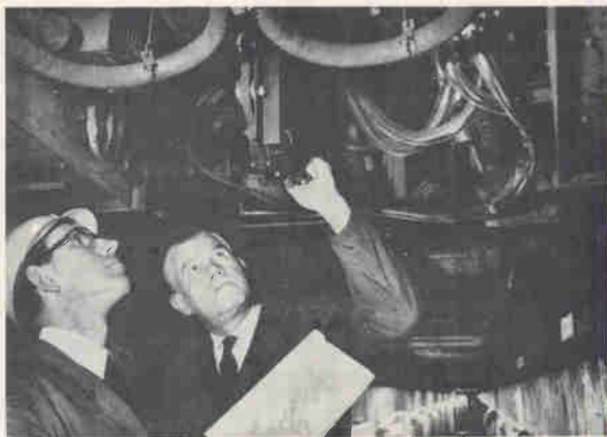
Looking up. Engineers inspect undercarriage of subway car on which is mounted Siemens coil antenna that detects crosspoints along the track.
