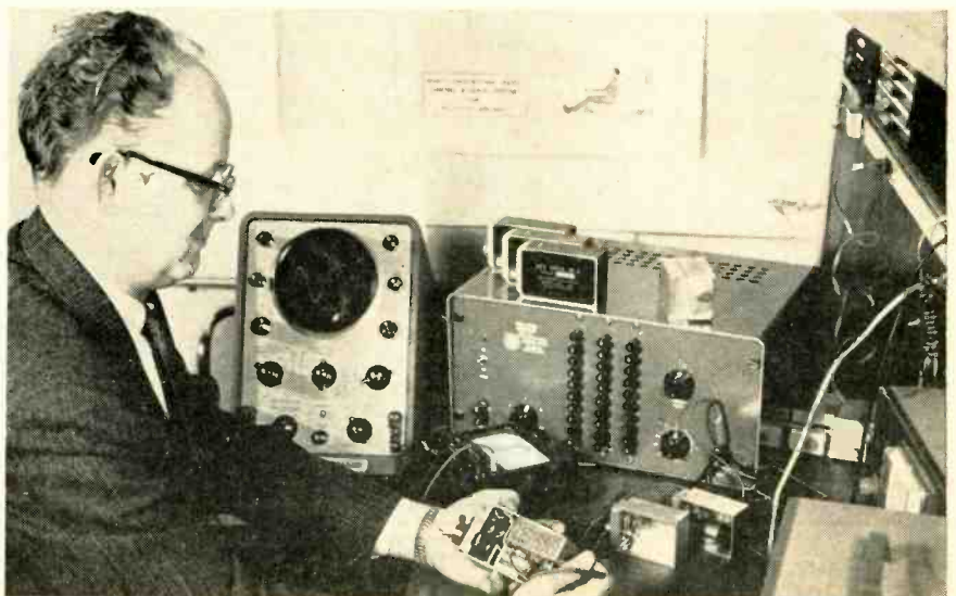
Measuring response characteristics of servo amplifier
