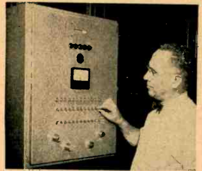
Newspaper mail room supervisor sets printing order on totalizer, waits for signal run is complete
