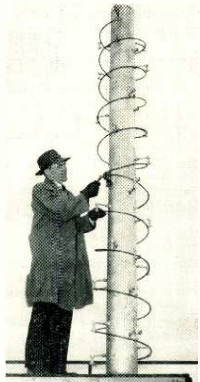
One of four sections of the side-fire helical antenna that provides a gain of 20 on the uhf television frequencies
