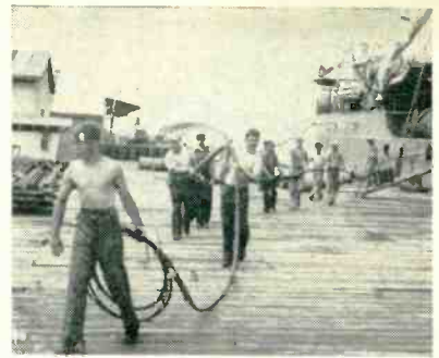
FIG. 1—Submarine cable repeater being taken off cable ship after laying tests
