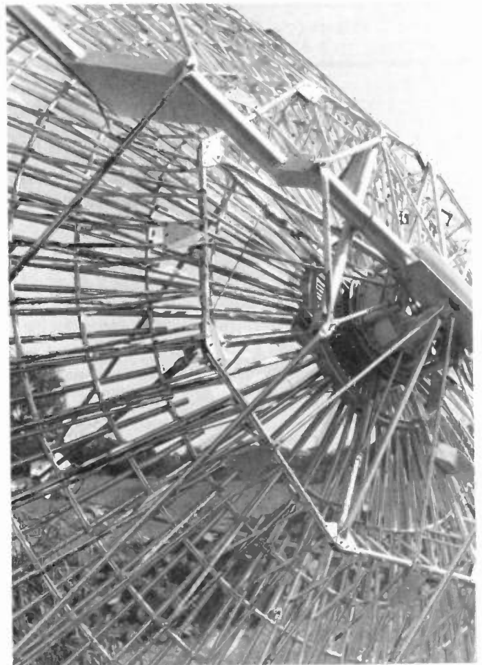
The dish, which is almost 16 feet in diameter, has a frame built from PVC pipe and electrical conduit. The supporting bar, which spans the dish, is the only piece that Tex did not fabricate himself.
