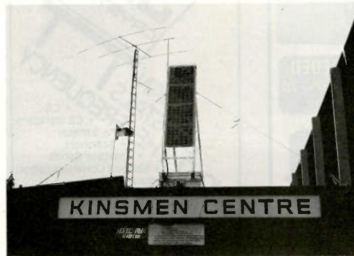
The power supply and tribander up on the roof of the exhibition building housing the station. The solar panels shown provided enough power to keep the six 105-Amp batteries stored at the base of the panels always close to full charge.
