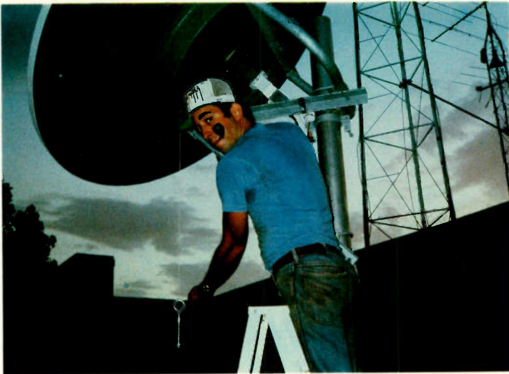
Photo H. The author checks the elevation angle on the six-foot satellite receive-terminal using a 29-cent protractor. The back of the dish presents a right angle to the feed, allowing use of a simple protractor with string and weight to check the elevation angle.
