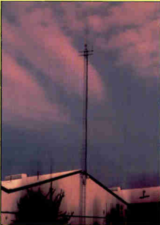
Here's an installation that is both unsafe—it's unguyed for more than 40 plus feet, and illegal because it's over 50 feet tall.
