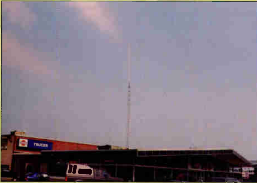
This CB dealership base antenna is a nice neat installation, approx. 40 feet tall and well-guyed.
