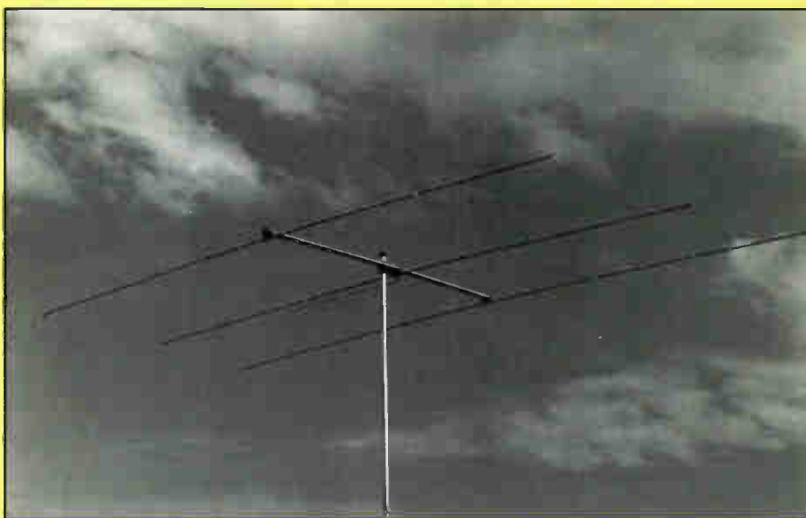
Always get a helping hand when installing ANY antenna. This large Cushcraft yagi is a snap to erect, as long as you plan your installation before "Antenna day." (Photo Courtesy Cushcraft Corp.)
