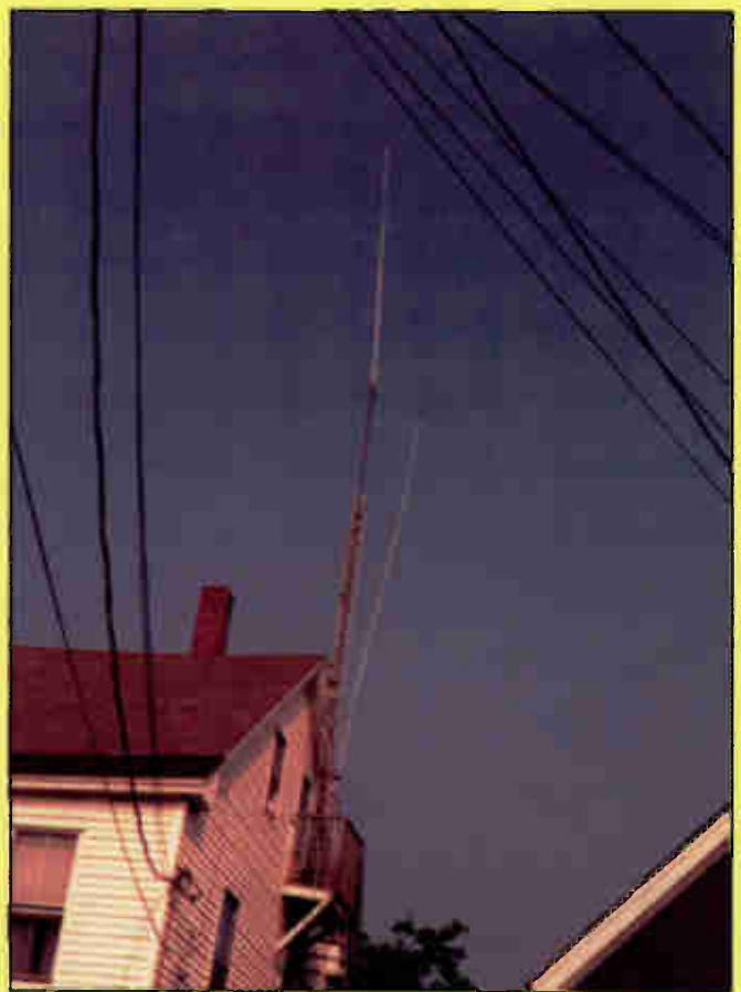
Here's a shining example of a poorly-maintained tower. It's completely rusty and has been erected too close to metal objects, including power lines. It's a disaster waiting to happen.
