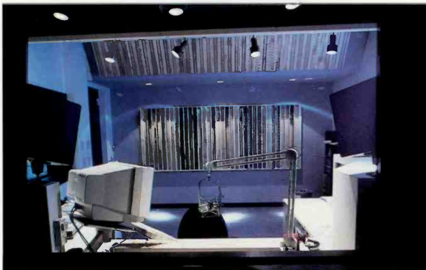
Looking into Control Room B from Studio B at Inter ocean Public Radio. Note diffuser panels on rear wall and ceiling section of control room.
