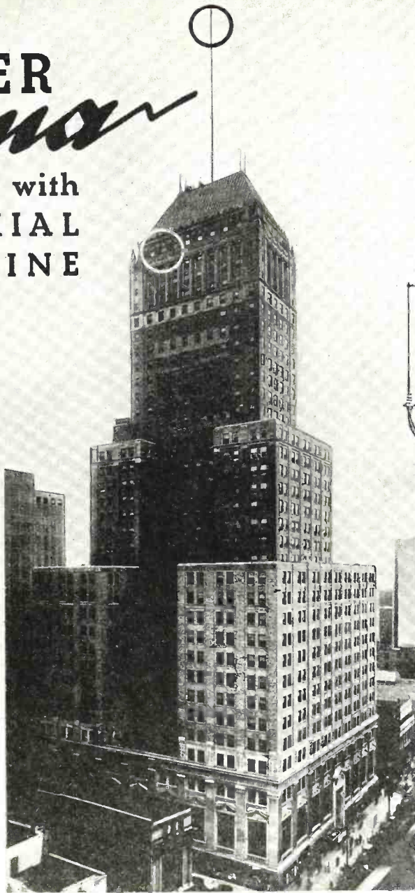
National Newark and Essex Bank Building. Showing location of transmitter and antenna connected by ISOLANTITE COAXIAL TRANSMISSION LINE.
