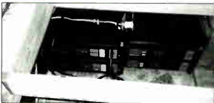
Three IT-1220's paired with three AR-1220 Voltage Regulators visible under the floor at Vital Recording.
