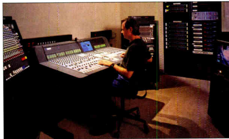
The Euphonix 2000B console and rolling equipment racks in the sound control center are linked to the Ghielmetti patchbay via Elco connectors. Meyer CP-10 equalizers and various delays occupy the permanent racks recessed into the control room wall.
