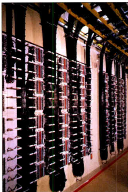
Microphone and line-level cross connect blocks
