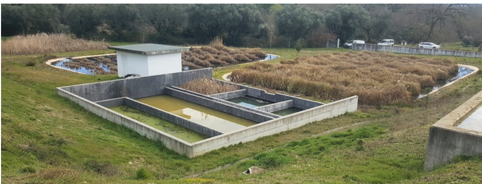
Fig. 4.3 Sedimentation and macrophyte basin and – no longer necessary – activated carbon filter bed and aerobic wetland at the Urgeiriça uranium mine, Portugal. Mine water ( Q \approx 90 \text{ L min}^{-1} ) flows from right to left, and pH is raised from about 6 to 8 on average. Iron, uranium and radium are retained in the system
