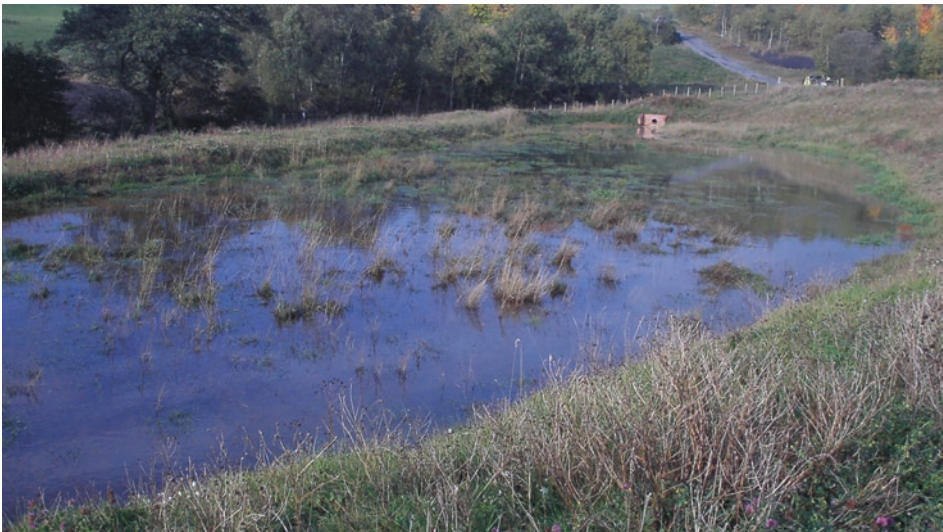
Fig. 4.14 RAPS II at the Bowden Close site, County Durham, England, looking west. Typical wetland plants are growing by succession on the substrate of limestone and horse manure. Outside the image on the right is RAPS I and on the left is the constructed wetland
