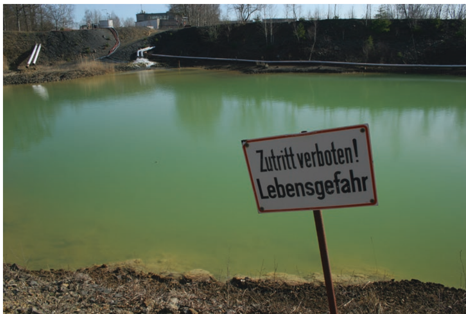
Fig. 4.15 Settling pond at the former Straßberg/Harz, Germany, mine water treatment plant. The green colour is mainly caused by suspended limestone. Since the relinquishment of this treatment system, the pond is overgrown with plants
