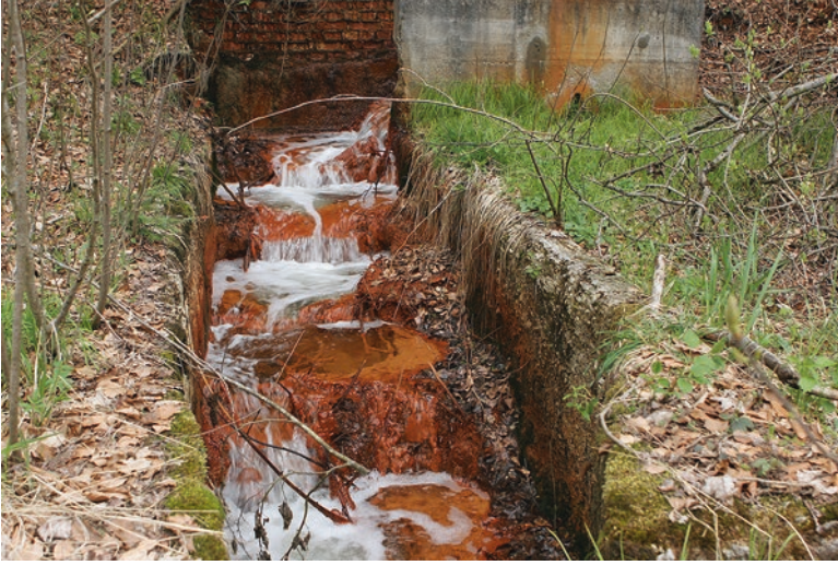
Fig. 4.21 Oxidation cascade of the ventilator adit on the Leitzach river, Upper Bavaria, Germany. Flow rate about 2 \text{ m}^3 \text{ min}^{-1} ; width of the channel about 1 m. In the meantime it was completely rebuilt
