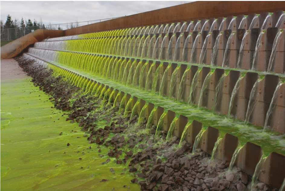
Fig. 4.22 Oxidation cascade of the Neville Street passive mine water treatment plant, Nova Scotia, Canada, during a tracer test with uranine (sodium fluorescein). Flow rate about 1 \text{ m}^3 \text{ s}^{-1} ; height of the individual cascade stages about 0.6 m
