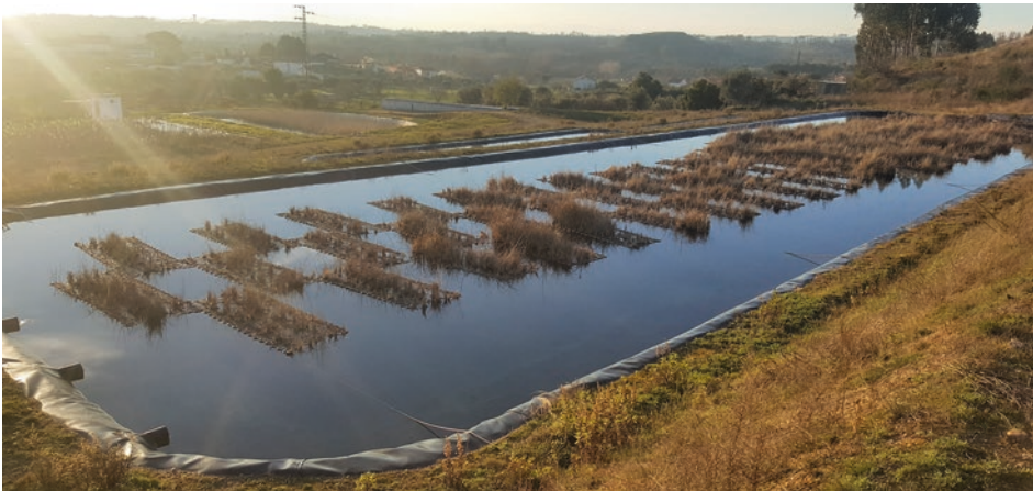
Fig. 4.26 Macrophyte basin of an ARUM system at the former Cunha Baixa uranium mine, Portugal. Iron, uranium and radium are retained in the system
