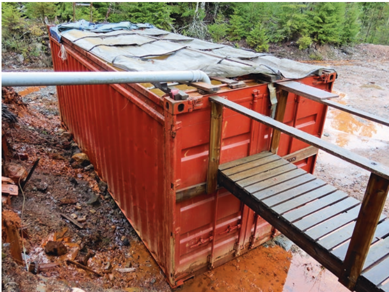
Fig. 4.20 Containerised vertical flow reactor (VFR) at the former Finnish polymetallic Metsämonttu mine with ventilation of the mine water (Sansox Oy OxTube). The outlet of the reactor with measuring weir for the flow is located at the rear end of the 20'-container (water volume: 24 m 3 )
