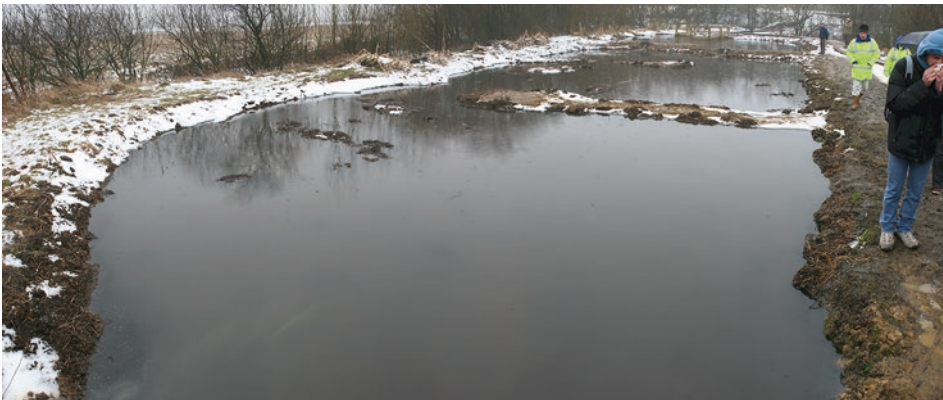
Fig. 4.8 First European anaerobic constructed wetland Quaking Houses (County Durham, England, United Kingdom). Plant cover is absent, as the sludge had been replaced after 10 years of operation
