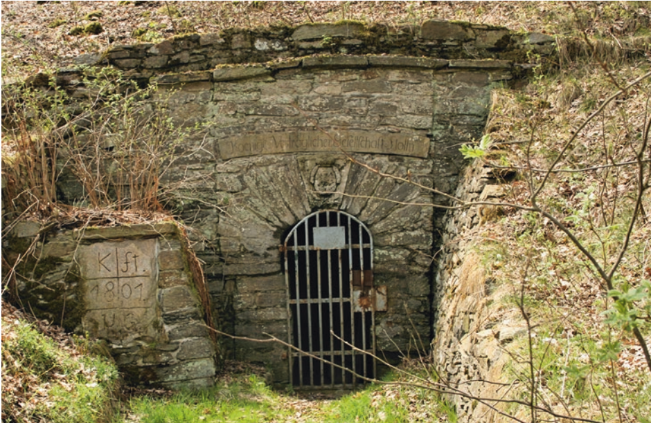
Fig. 6.10 “Königl. Verträglicher Gesellschaft Stolln” at the Rote Graben near Freiberg/Saxony, Germany, from the nineteenth century, closed with a grid. Part of the World Heritage Site Montanregion Erzgebirge/Krušnohoří
