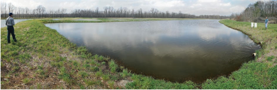
Fig. 4.1 Part of the passive mine water treatment system for the tailings pile at Enos Colliery (Pike County, Indiana, USA). The operation of the wetland is described in Behum et al. (2008). (The photo composite shows the Canal Aerobic Wetland in the 6.5 ha constructed Enos East wetland)
