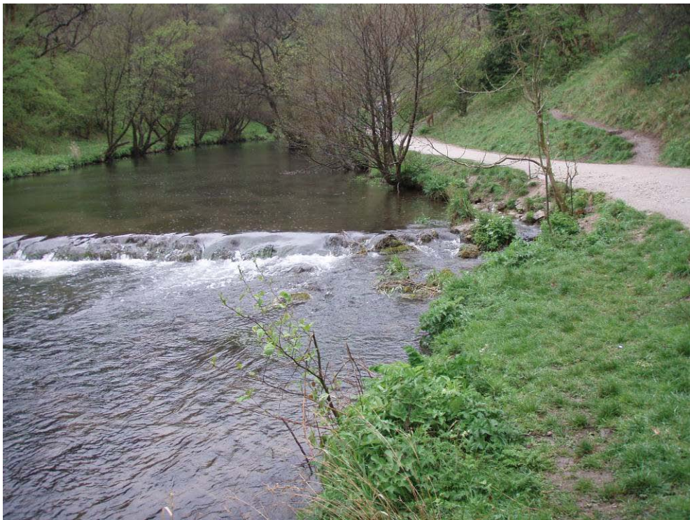
Photo 4 Impounded section above a weir – slow-flowing, uniform and now relatively wide and shallow – the opposite of the original intended effect of the weir?
