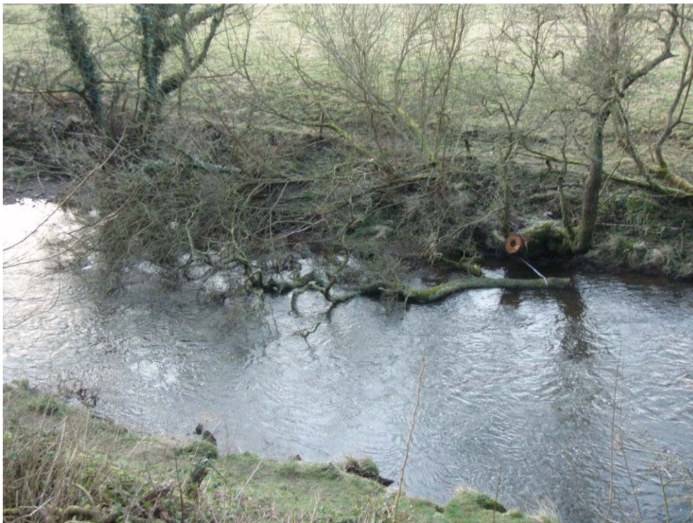
Photo 9 Introduced LWD on the River Manifold
