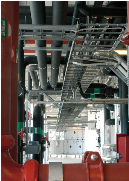
Wibe Cable Ladder KHZP installed at Kista Science Center, Sweden.
