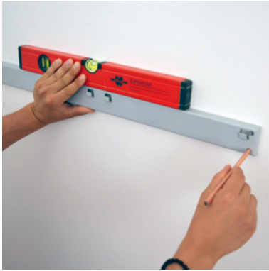
Mark drill holes
