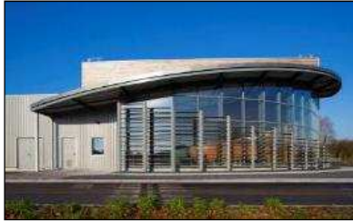
Usine eau potable
