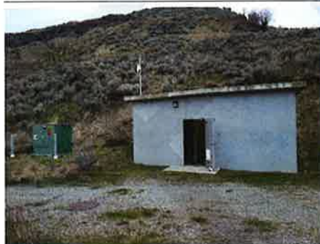
The Rise Booster Station
