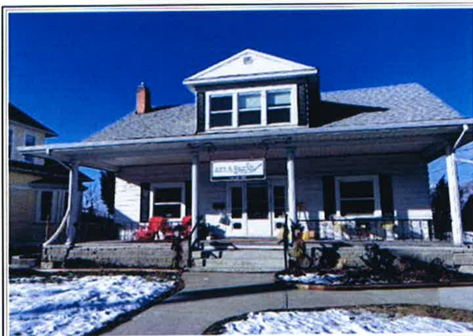
(BELOW) Photo from appraisal document shows inappropriate alterations made by previous owners – including: metal siding, 'Grecian' columns, & iron porch railings.
