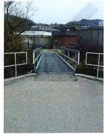
Vehicle Access Bridge
