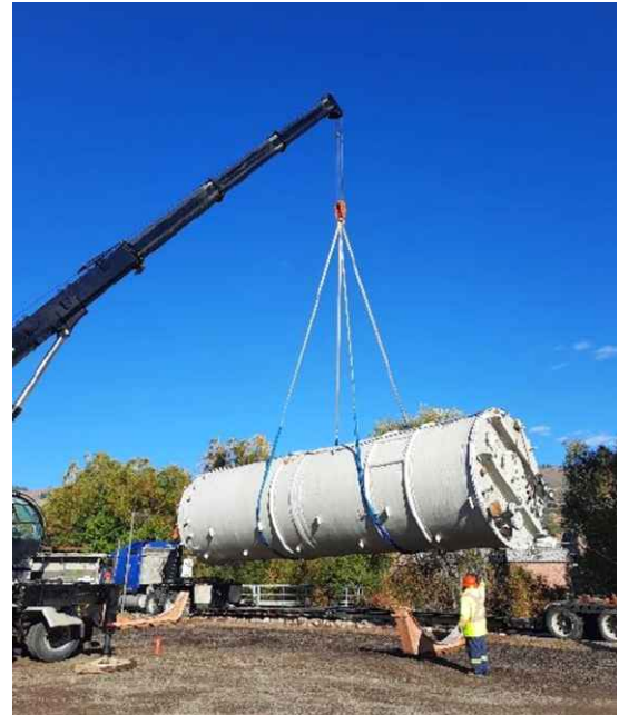
Staff unloading HRAD facility reactor tank.
