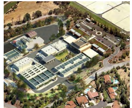
RWTP Reliability Improvement
