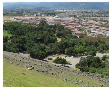
Anderson Dam during DSOD inspection
