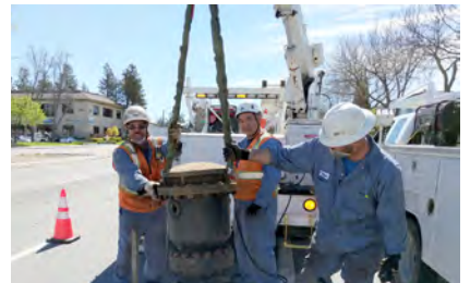
Parallel East Pipeline Refurbishment
