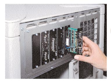
APC's line of award-winning SmartSlot accessories slide right into the back of Symmetra, and integrate with PowerChute products or PowerNet SNMP management software to communicate necessary information and commands.
