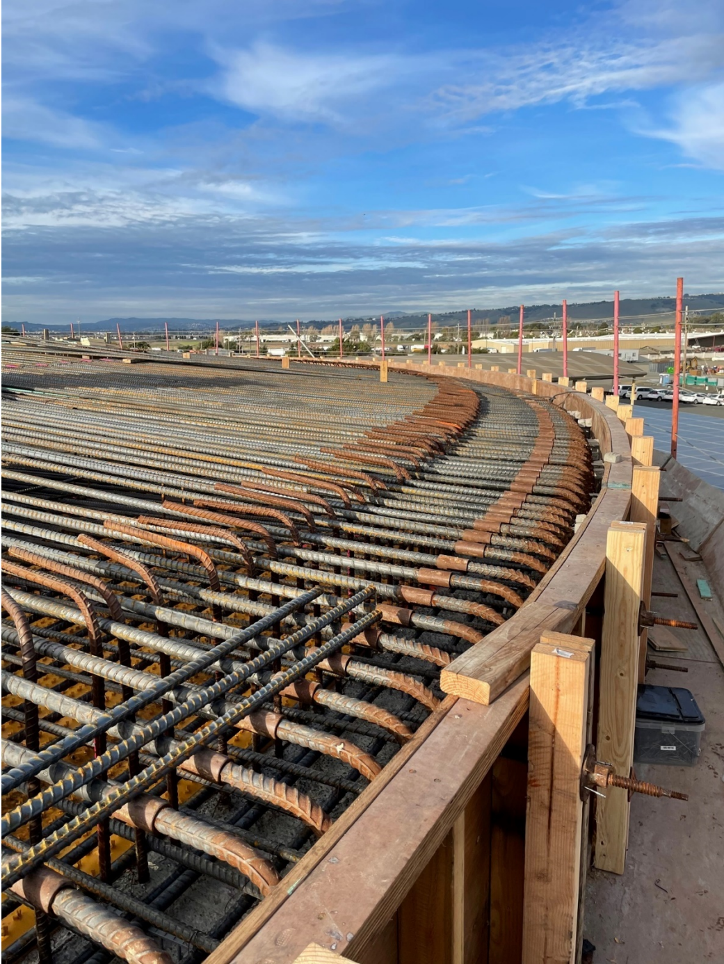
Rebar Layout Digester 7 Roof
