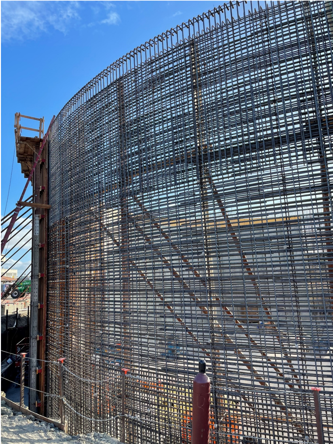
Digester 7 Wall Construction
