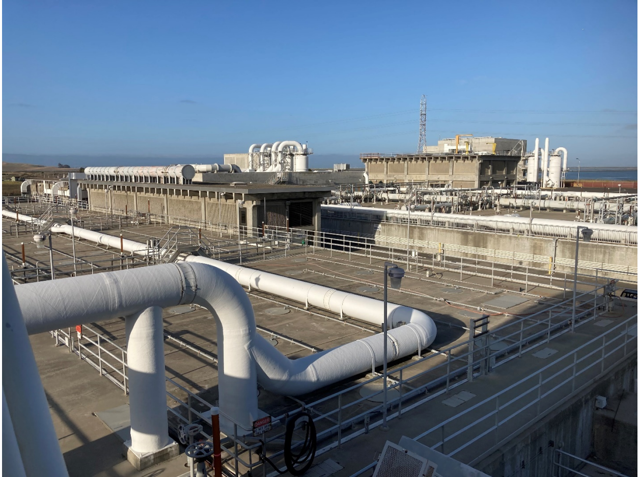
Looking West Across the Aeration Basins
