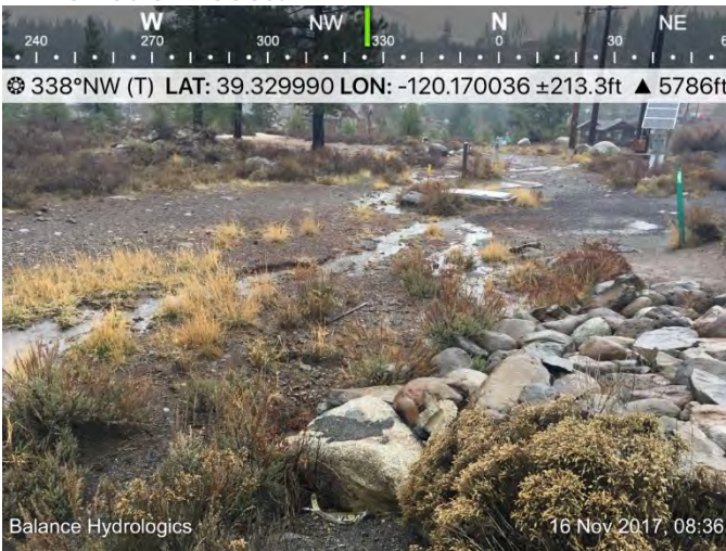
Figure 3-4. Sub-Watershed 17: Concentrated Stormwater Runoff Leading to Erosion in an Area with No Stormwater BMPs.
