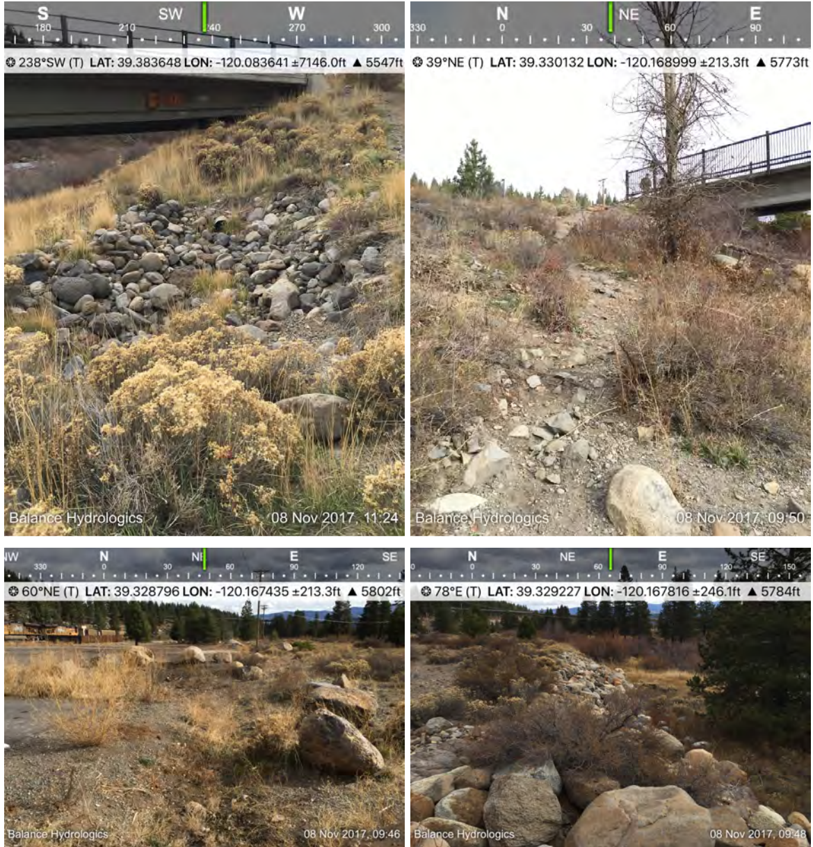
Figure 5-8 Legacy Trail Bridge Existing Site Conditions. Top-left: Fill and vegetation stripping near bridge. Top-right: Erosion from makeshift public access trail. Bottom-left: Existing stormwater detention basin. Bottom-right: Fill material.
