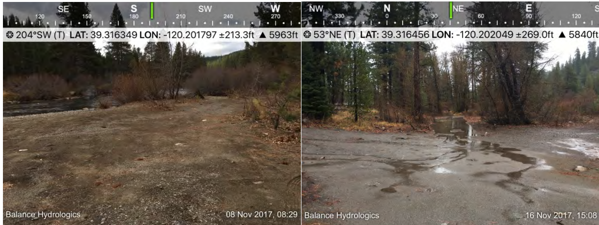
Figure 3-9 Donner Creek Confluence. Left: Compacted Soils Along Floodplain. Right: Stormwater Runoff from a November 2017 storm.
