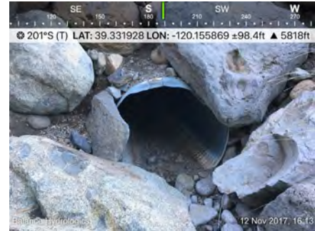
Figure 1-1. Example: Sediment Conveyance by Stormwater Infrastructure (Legacy Trail by Truckee River Regional Park)
