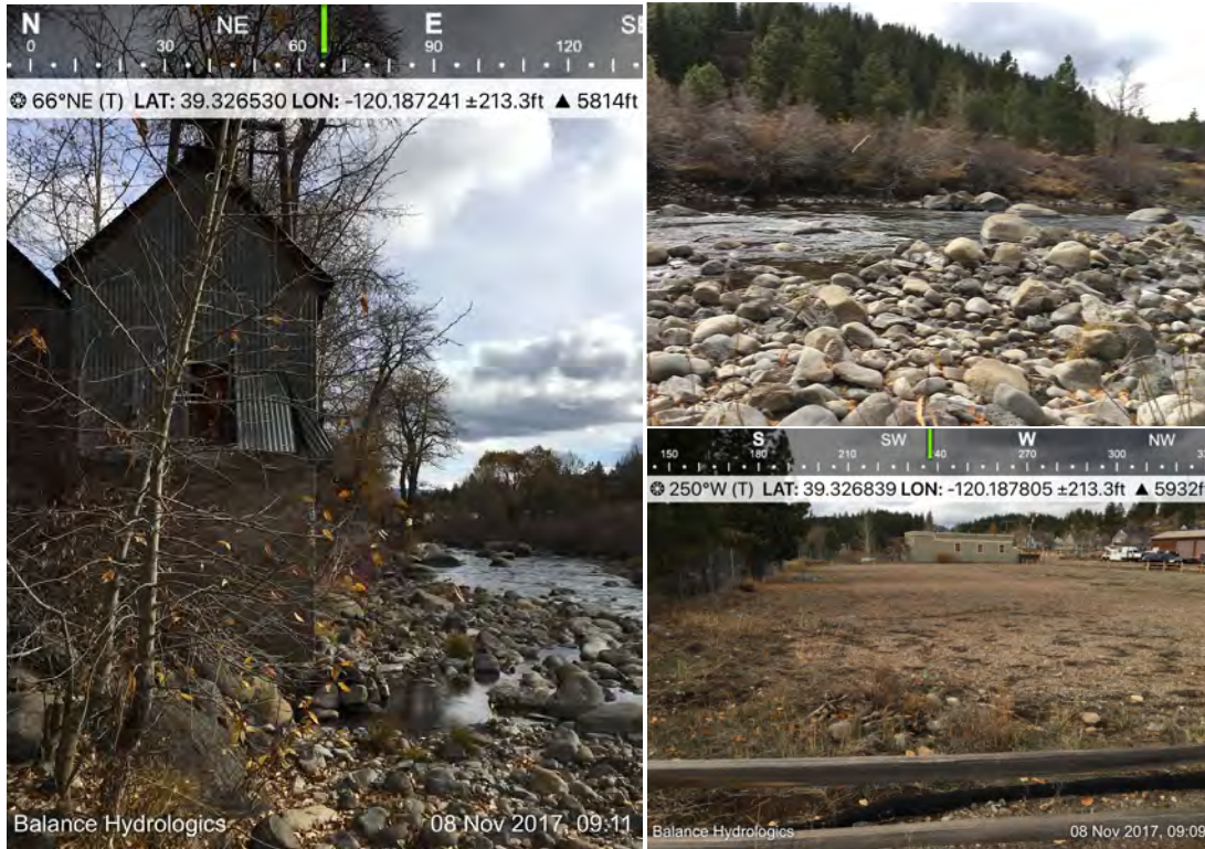
Figure 5-4 Riverside Drive Bridge Crossing Site Existing Conditions. Left: Historical building that could be preserved. Top-right: River access location. Bottom-right: Fill at river left bank, area of the old corps yard. PR-4: Truckee River Regional Park Riverside Parking Area
