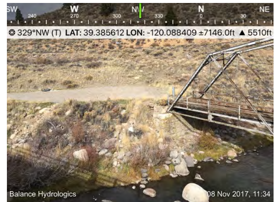
Figure 1-3. Example of a Historical Site and River Access Location, Boca Bridge.
