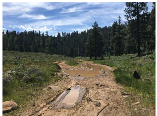
Vehicular access routes compacted soils and divert runoff to the Truckee River
