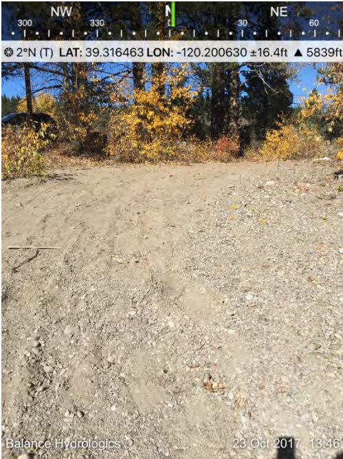
Figure 3-2. Sub-Watershed 1: Disturbed Sand Bar on Floodplain from Vehicular Access.
