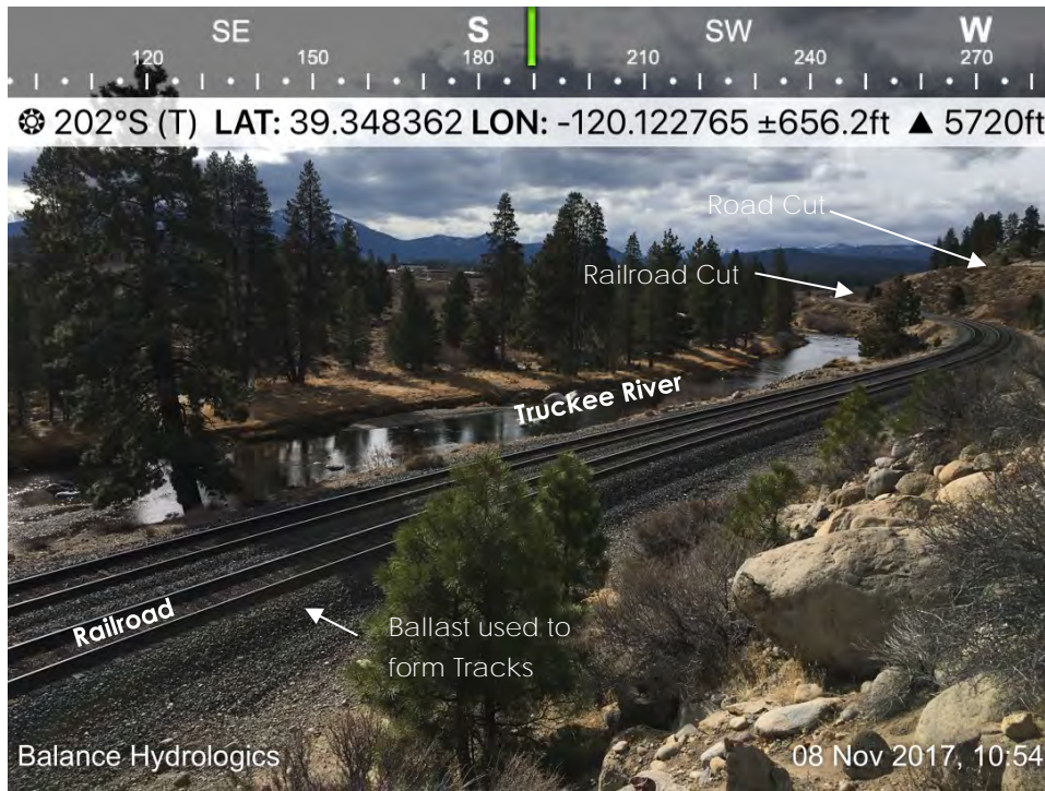
Figure 2-13 Examples of Railroad Features Impacting the Natural Hillslopes and Introducing Sediment Sources to the Truckee River. Near Glenshire Drive Looking West Towards Town of Truckee.
