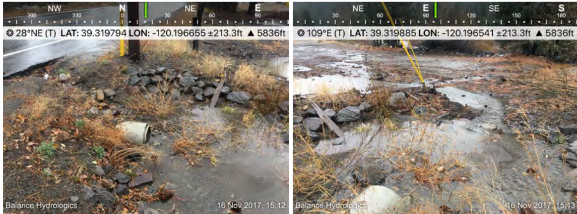
Figure 5-3 Donner Creek Confluence Site Existing Conditions. Left: Sediment basin at base of stormwater culvert at filled with road sand. Right: Runoff leaving basin and picking up sediment through parking area.
