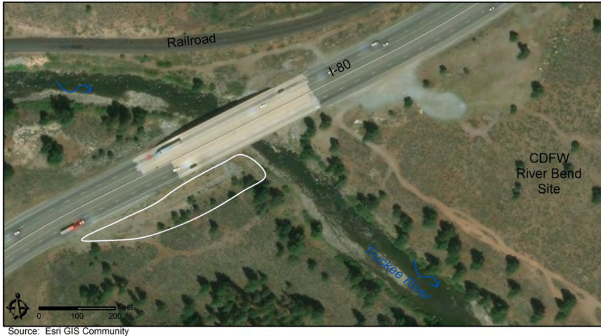
Figure 5-14 I-80 Bridge Stormwater Erosion Potential Restoration Area.
