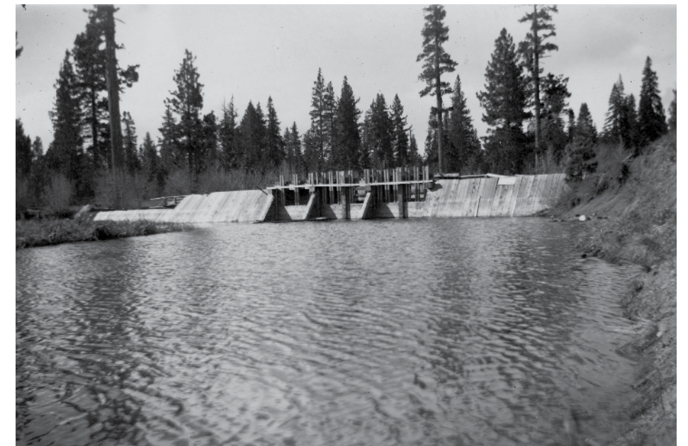
Timber crib dam, (early 1900's) — Special Collections Department, University of Nevada, Reno Library
