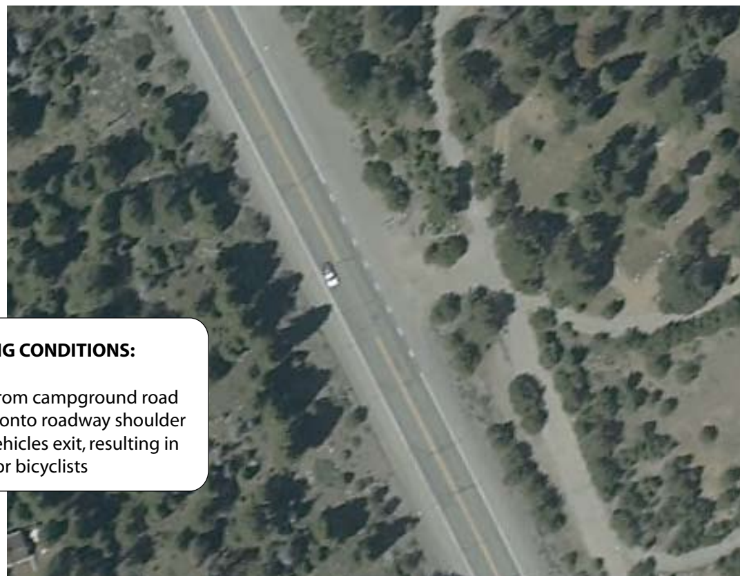
EXHIBIT 4-20 Silver Creek Campground Exit Road Improvements
