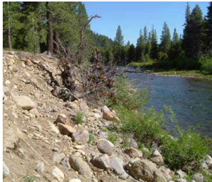
5. Eroding bank with downed trees and in-stream woody material
