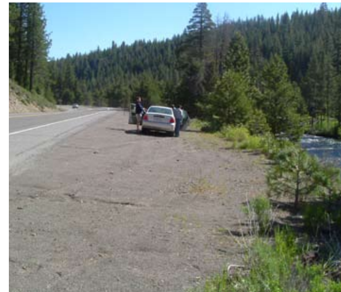
11. Wide unvegetated shoulders could accommodate a Class I trail or should be revegetated to reduce sediment into Truckee River
