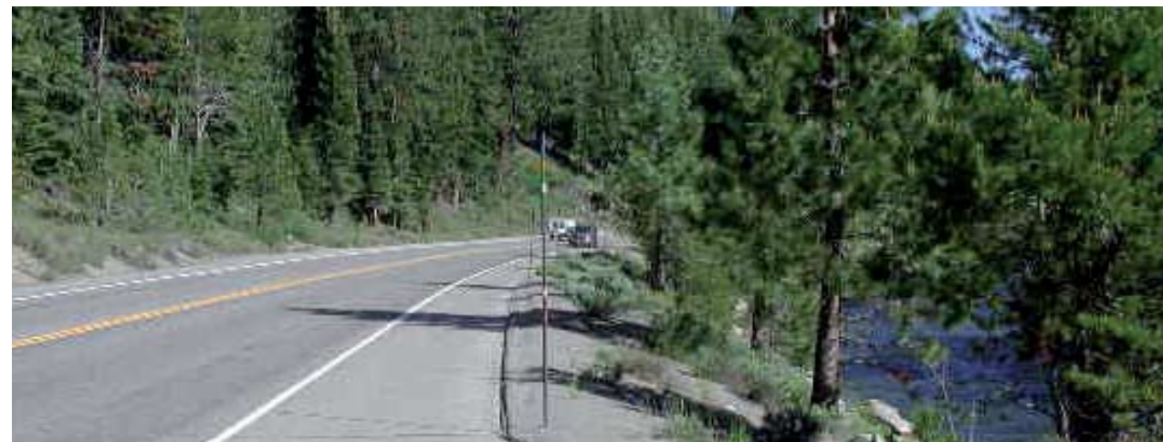
Existing shoulder bike lane adjacent to roadway, 2005
