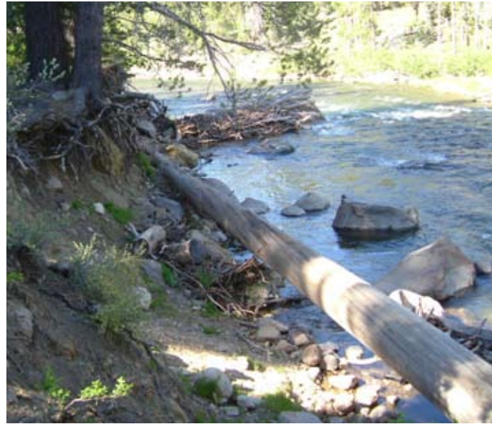
7. Heavy bank erosion and woody debris
