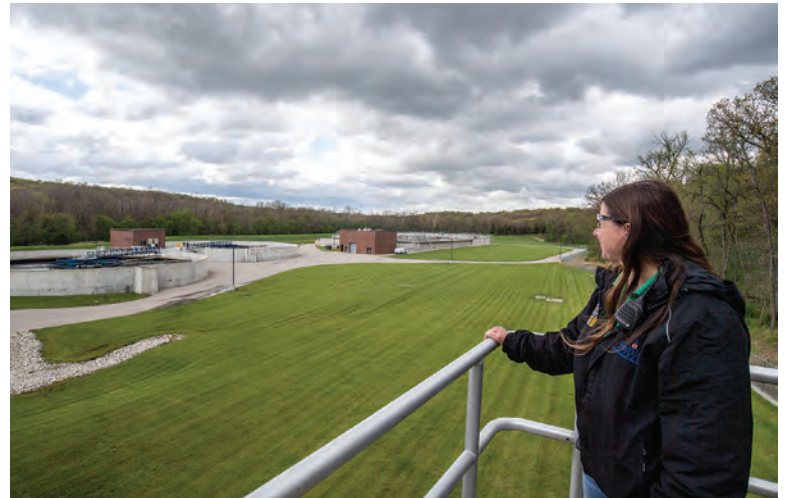
Phillips oversees a 7.75 mgd (design) facility that uses a process developed by biological nutrient removal pioneers.
