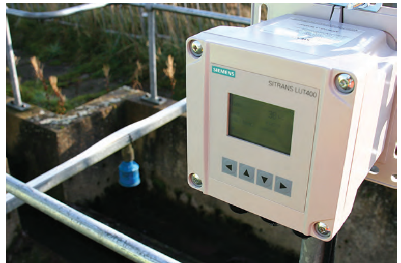
An ultrasonic controller and transducer interfaced by way of a transducer cable.
