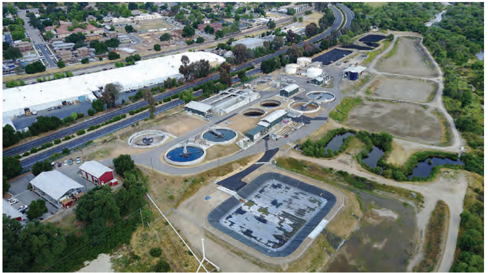
The Paso Robles (California) Wastewater Treatment Plant has a design capacity of 4.9 mgd and an average flow of 1.9 mgd.
