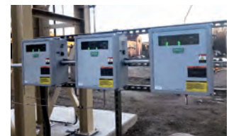
H2S Scrubber Monitoring System from MSA Safety
