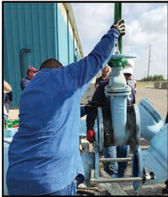
Spread outside flanges & remove old valve
