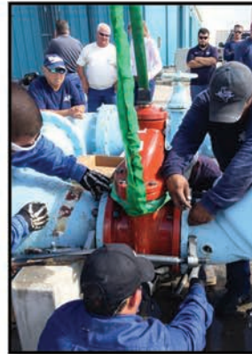
Reinstall new valve
