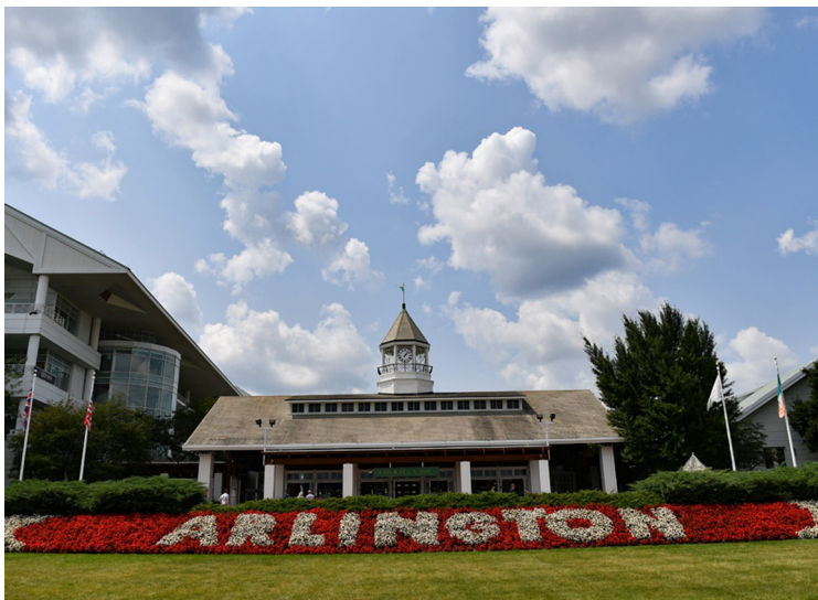
The grandstand entrance at Arlington Park | Horsephotos
