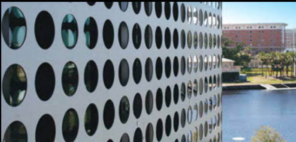
Nearly 3,800 panels of McNICHOLS® Perforated Metal, Aluminum Type 5005-H34, Anodized, .125" Thick, 3" Round on 4" Straight Centers, 45% Open Area, were used to create a facade for the Tampa Museum of Art.
