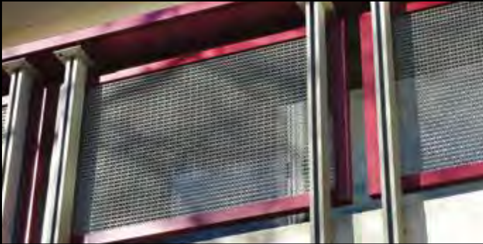
McNICHOLS® Designer Wire Mesh, TECHN ™ 3156, Stainless Steel Type 316, 61.2% Open Area, was specified for railing infill panels on the balconies of this Providence, RI, housing development.
