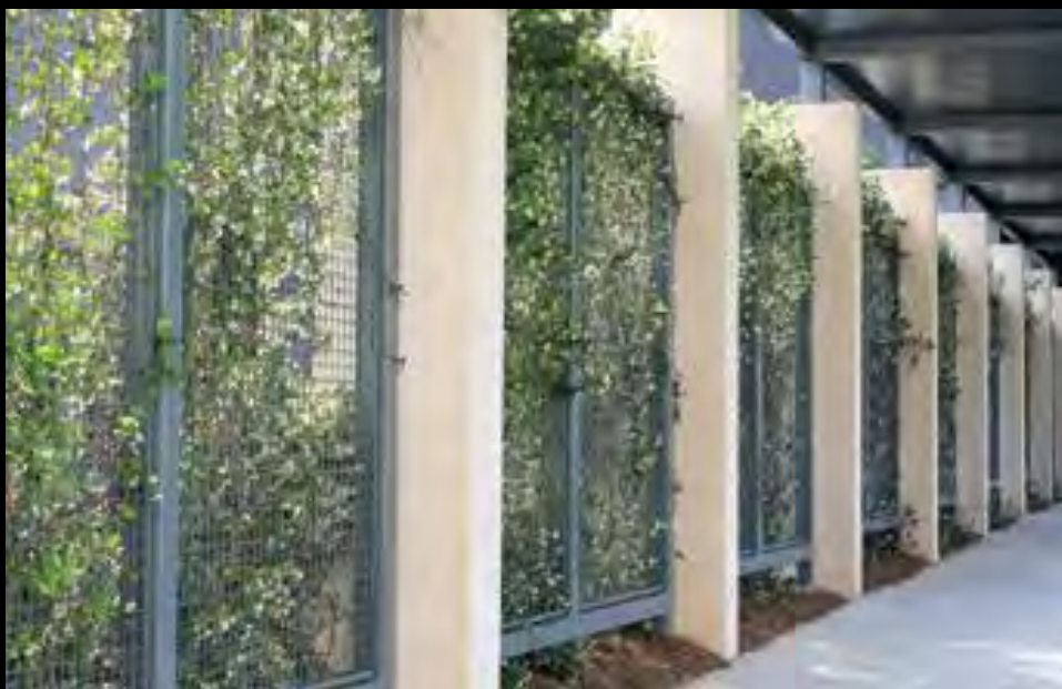
McNICHOLS ECO-MESH® Modular Trellis System was selected to add beauty and shade to a walkway at the H. Lee Moffitt Cancer Center's McKinley Outpatient Center in Tampa, FL.
