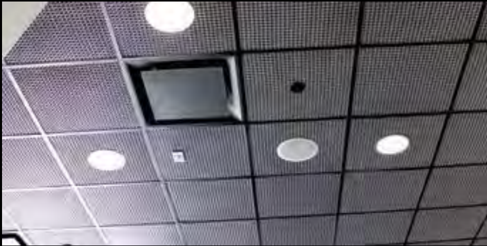
McNICHOLS® Designer Wire Mesh, TALICA™ 8146, Stainless Steel Type 304, 61% Open Area, ceiling tiles overlook the entryway of an art and design school in St. Louis, MO.
