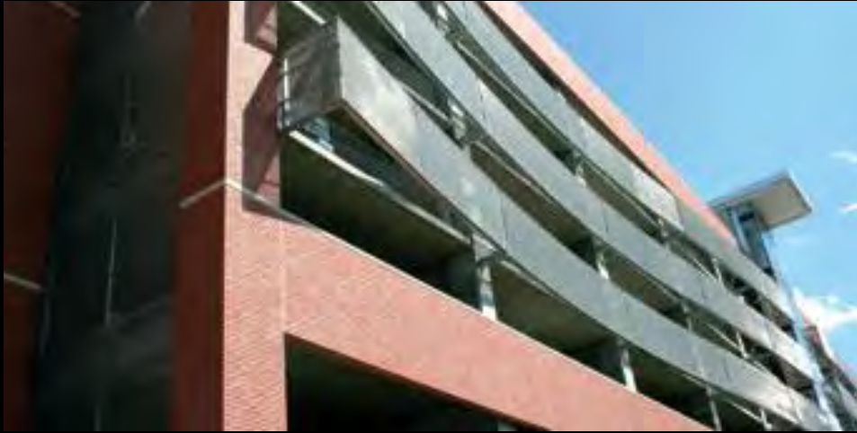
McNICHOLS® Designer Wire Mesh, CHATEAU™ 3105, Stainless Steel Type 304, 58% Open Area, used on this parking garage, adds beauty while allowing for passage of air and light.
