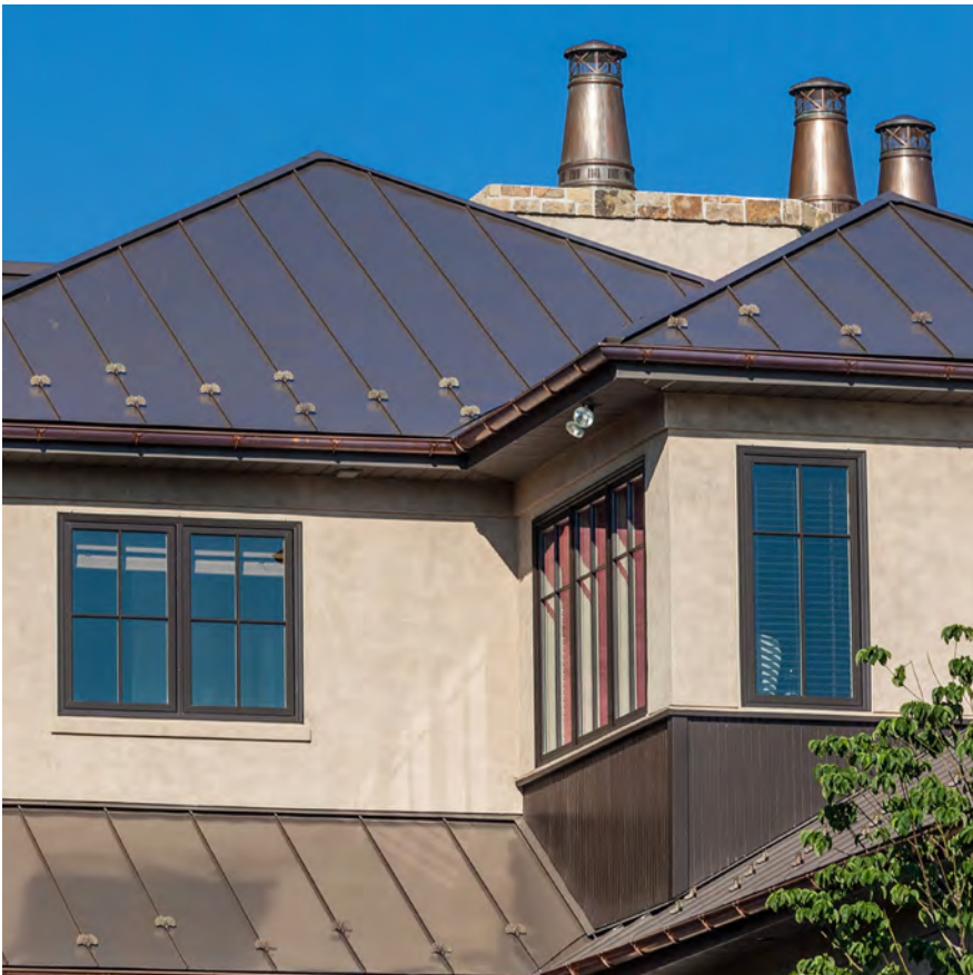
This home features a standing seam roof with Chimney Pot accents and a Snow Retention System.
