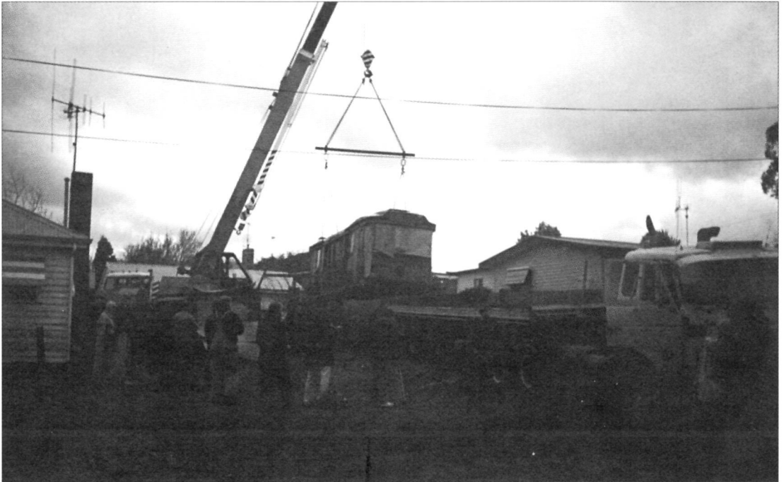
Car 22 is lifted from its resting place at Golden Square on 14 June 1995 for transport to the Gasworks Depot for safe storage and eventual restoration.
