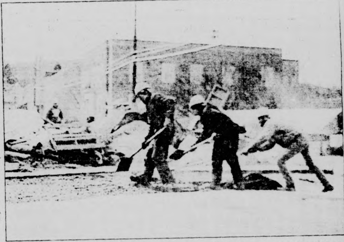
MEN AT WORK PAVING THE SURFACE of the Fourth Street railroad bridge in Emmaus, which is now expected to be completed by Jan. 13.
