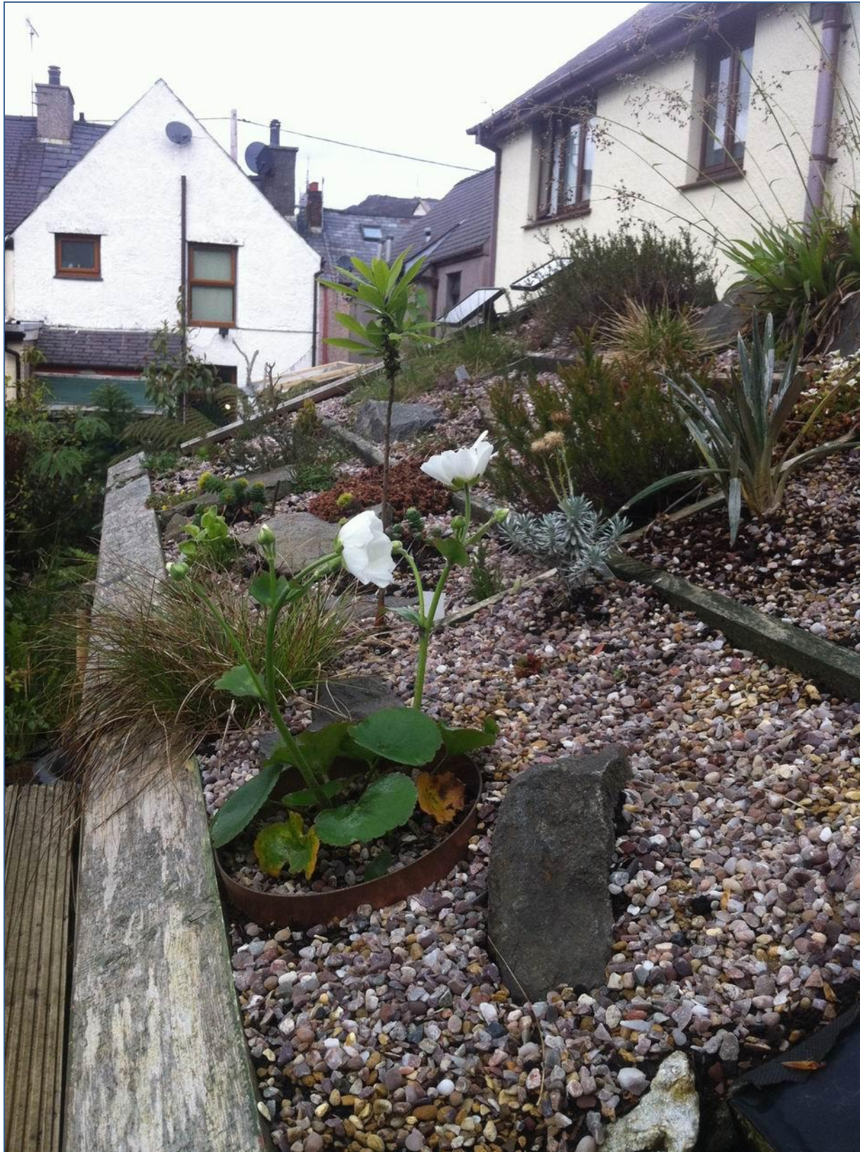
Overview of the shed roof - showing the wooden grid system, photo R.B-M.
