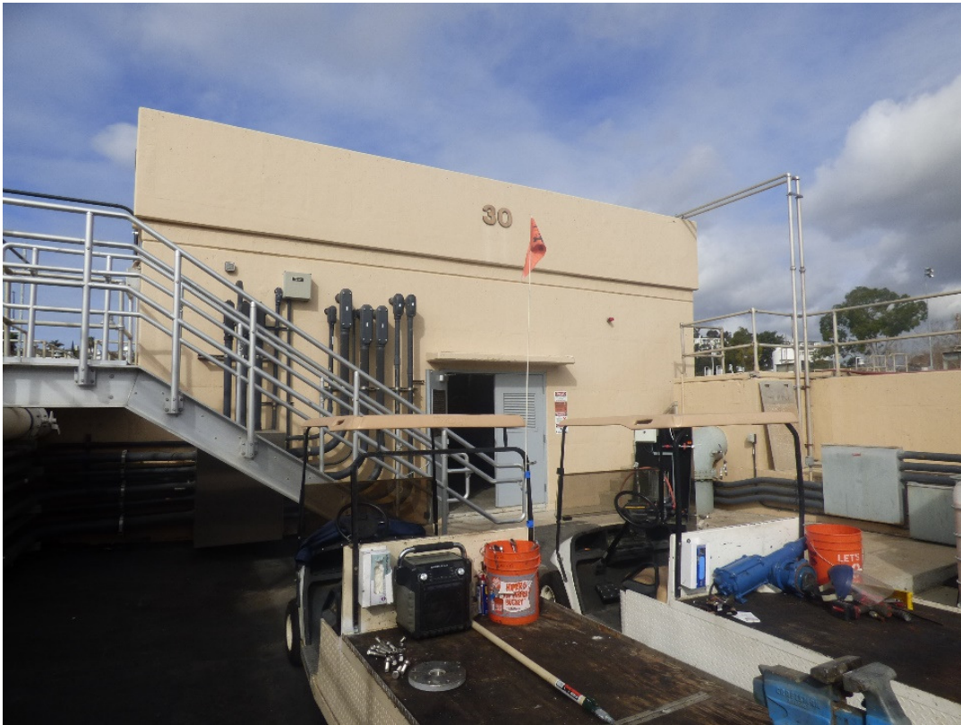
View of Plant 1 Blower Building (view to northwest)
