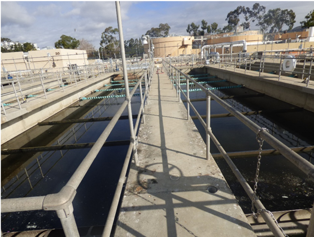
View of Secondary Clarifiers
