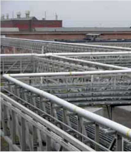
Wibe Cable Ladder KHZV installed at Outokumpu Stainless steel, Avesta Sweden.
