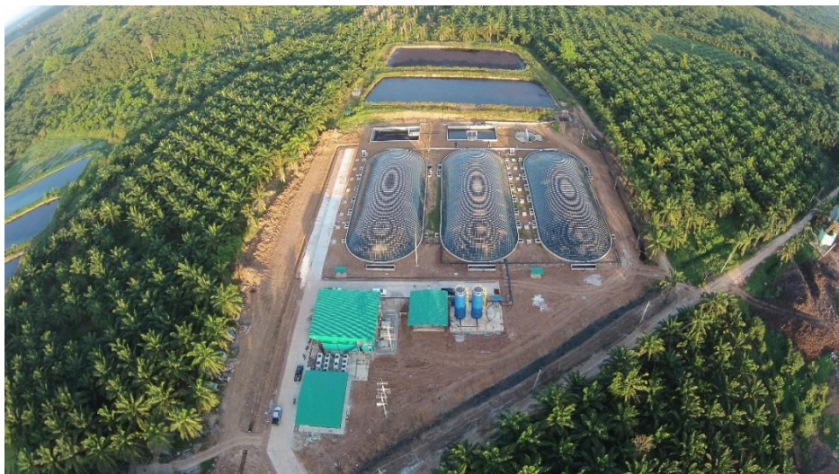
Biogas pond, Phrasaeng Power Plant, Surat Thani Province
