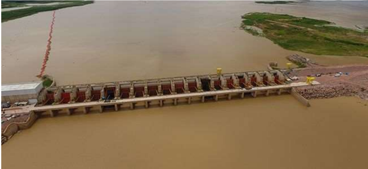
Fig. 1 Jirau run-of-river hydropower project. Sluice gates on the right side.
