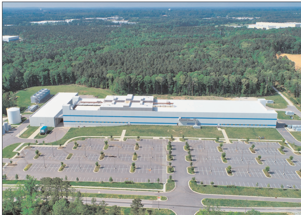
A five-year investment will leverage Cree's North Fab building and refurbished 200mm equipment to yield an automotive-qualified production facility.
