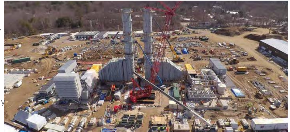
State-of-the-art peaking plant under construction at Medway.
