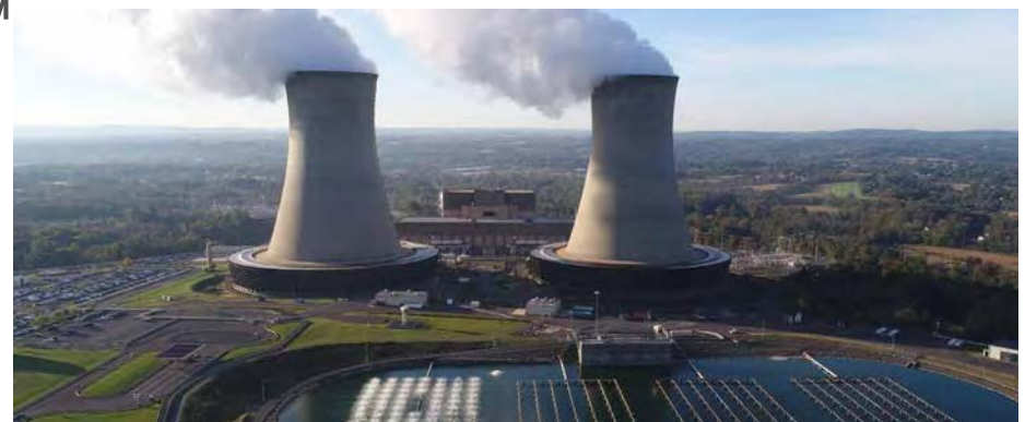
The Limerick Generation Station, located on the Schuylkill River in Pennsylvania, uses cooling towers to reduce the volume of cooling water needed.
