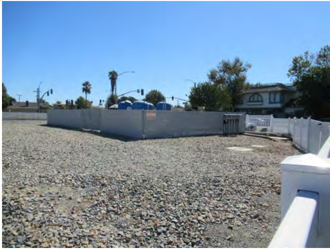
Looking South from Western Project Edge
