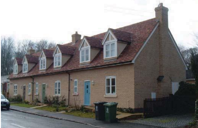
Infill development in Madingley designed to be sympathetic to the scale and form of its village setting.
