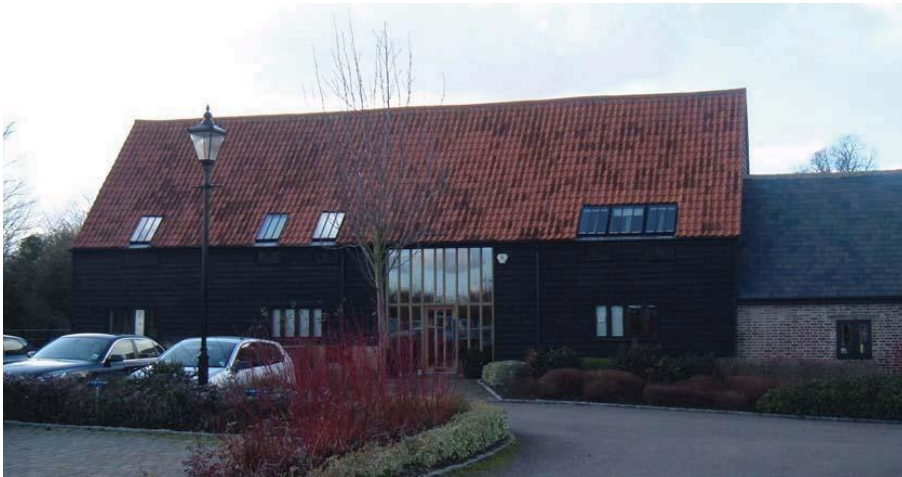
Kings Road, Hardwick, view of the main barn from the car park.
