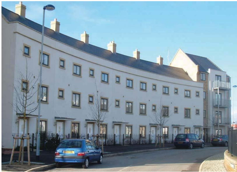
The size, shape and alignment of windows on a plain background of the building elevation, creates a primarily horizontal emphasis, giving the impression of a long low terrace. Orchard Park.
