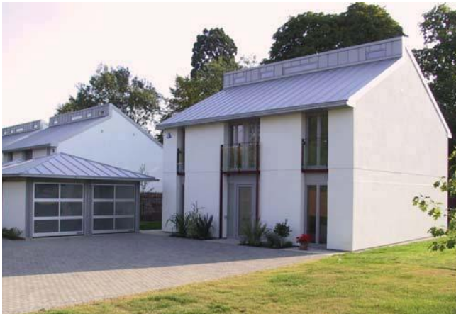
Infill houses, Melbourn. The rendered walls and tall window proportions make reference to the listed house, with contemporary metal roofing and window frames (Plum Developments).
