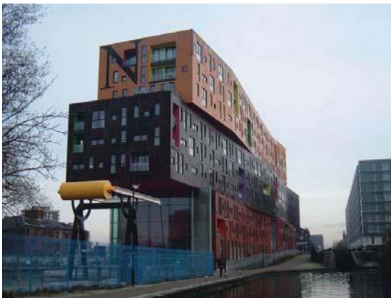
An innovative approach to the form of a building creates the visual impression of 3 separate forms stacked one on top of the other. The CHIPS building New Islington, Manchester.
