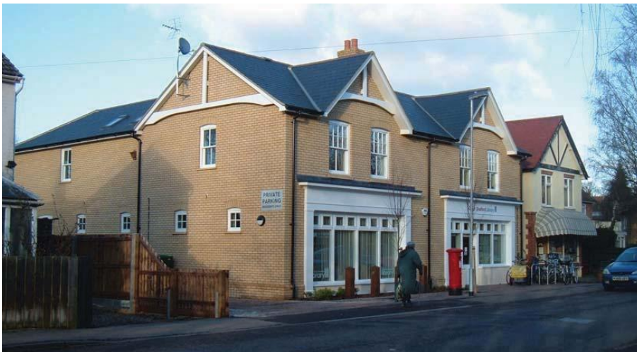
Great Shelford library with residential development above.
