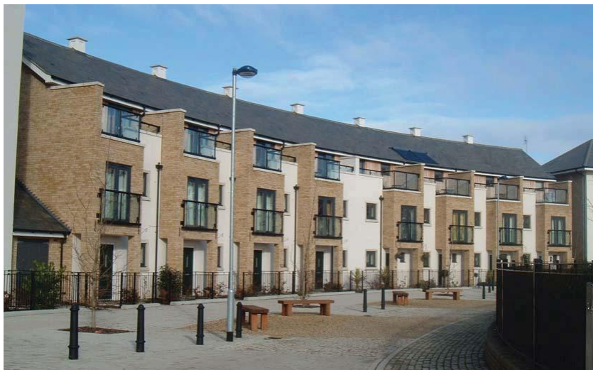
Vertical bays on similar terrace to the one above, creates a primarily vertical emphasis, giving the impression of a shorter and taller terrace than the one above.
