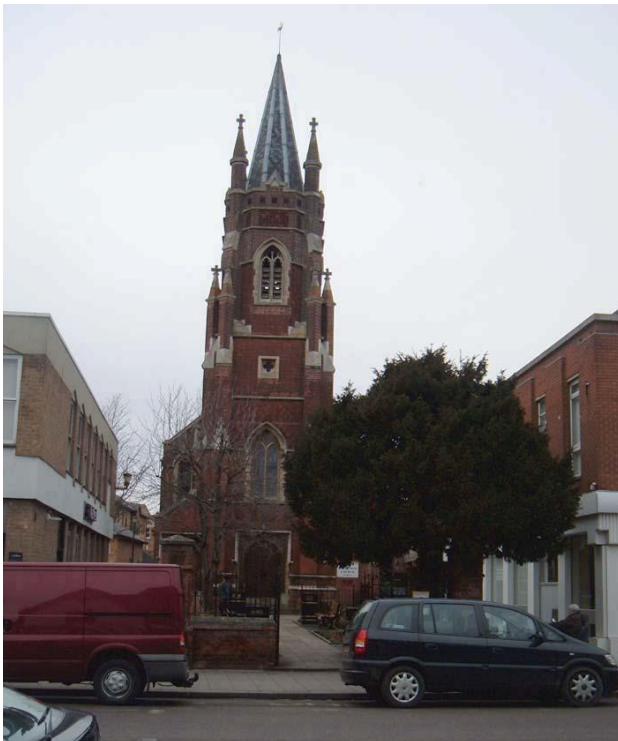
7. On the left hand side an opening in the built form fronting the street provides a view of the second church front with its spire.
