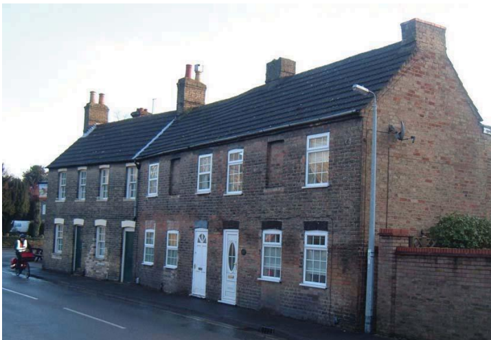
Blind windows used to continue the rhythm of openings in the façade of a terrace. St. Neots.
