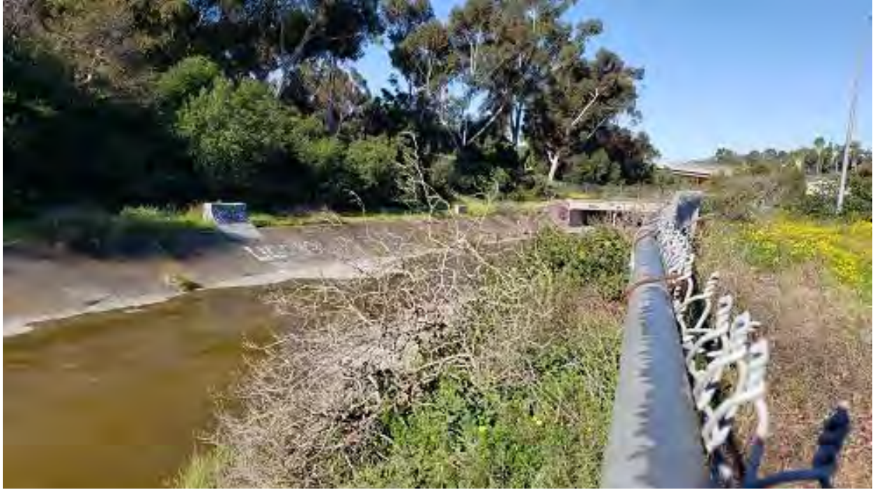
Photo 5. View of Chollas Creek looking downstream, near lower reach.
