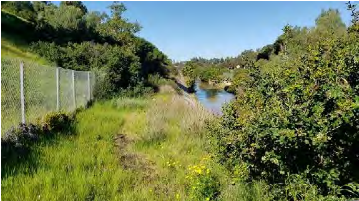
Photo 10. Same location as Photo 9. Retaining wall will be constructed just to the right of the fence to the SR-94 Caltrans slopes. Looking downstream.
