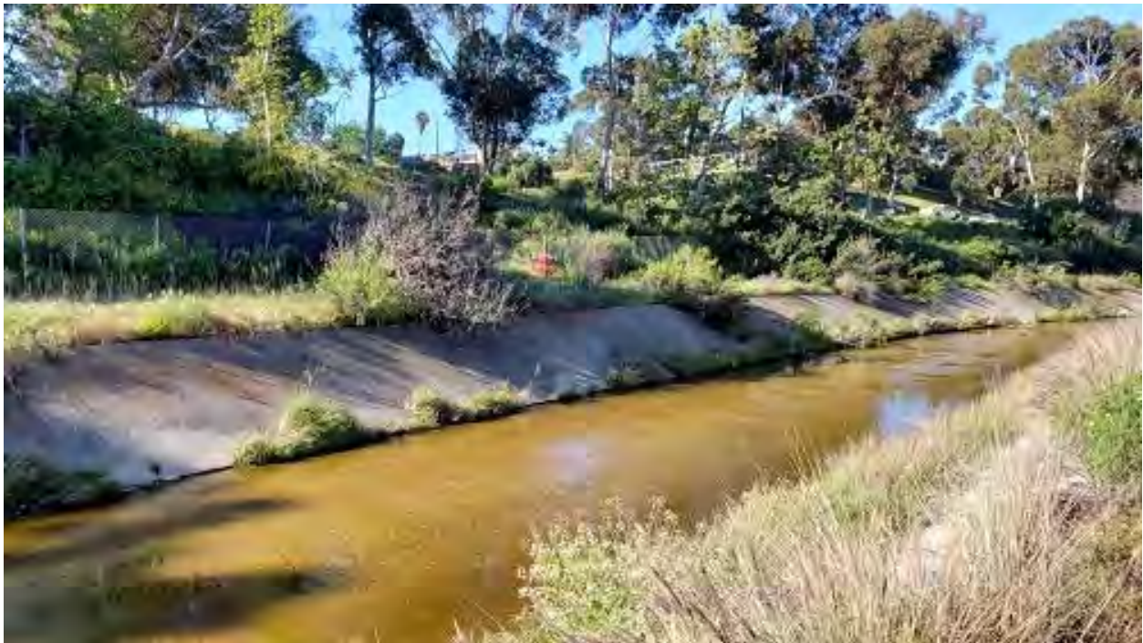
Photo 6. Photo taken just after rain. Flat disturbed area above concrete and in front of Caltrans chain link fence will be the location of the proposed retaining wall. Looking downstream.
