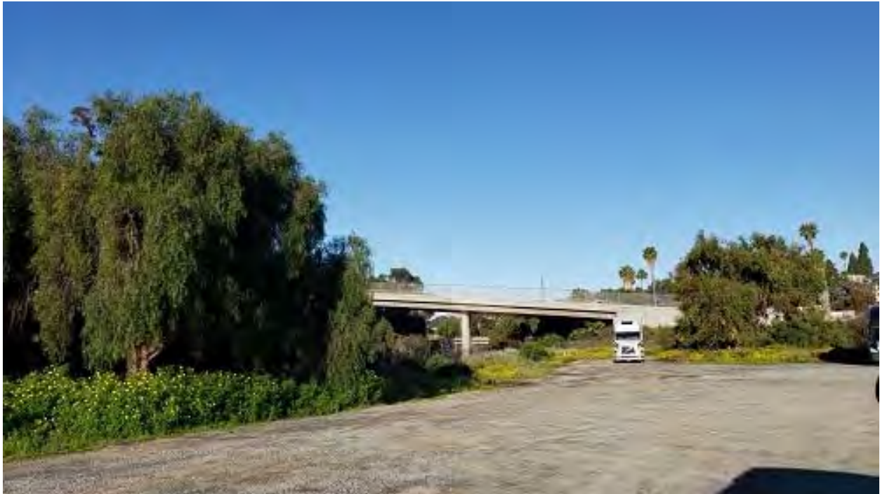
Photo 3. View of staging area near Home Avenue. Looking west.
