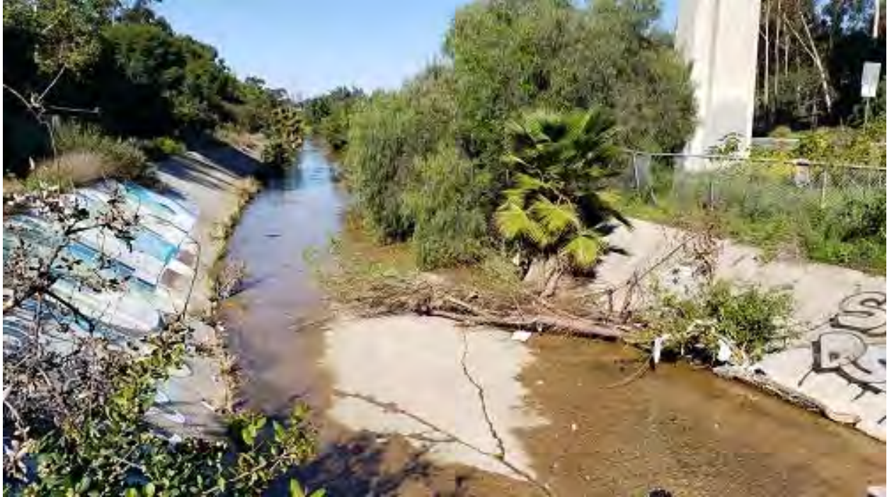
Photo 9. View looking downstream at upstream-most section, at culvert. Concrete channel will remain on the initial 80' to just past I-805 bridge pillar. Peruvian peppertree and Mexican fan palm are rooted in uplands above the channel.
