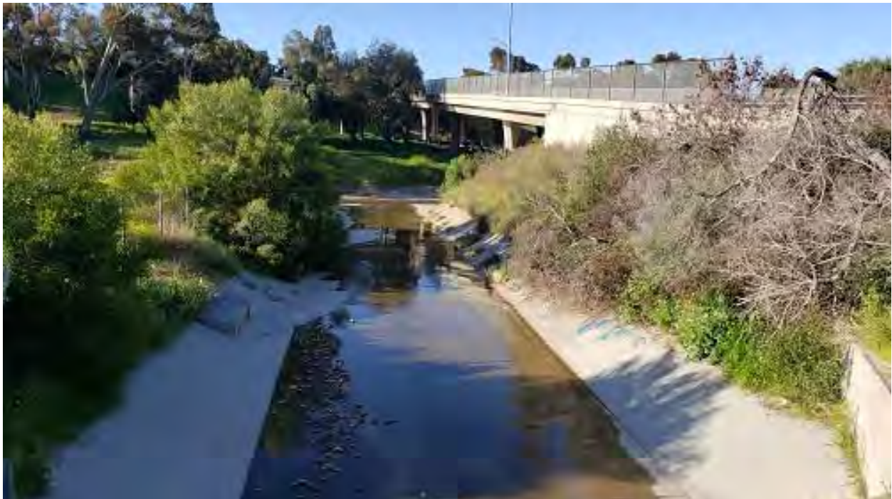
Photo 2. Side tributary coming into Chollas Creek that will remain in place.
