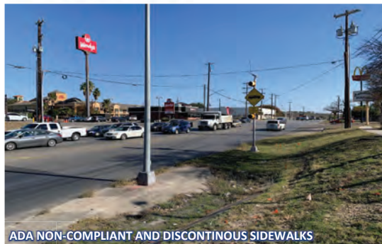
ADA NON-COMPLIANT AND DISCONTINUOUS SIDEWALKS
