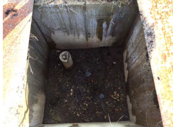
Photograph 4-2. Well Pit (Internal)
