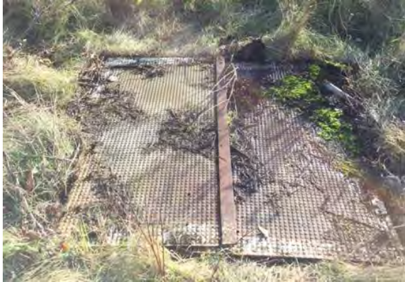
Photograph 4-1. Well Pit (Covered)
