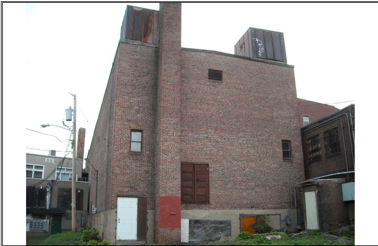
Photo 2: North-looking view at the back wall of the Site building.
