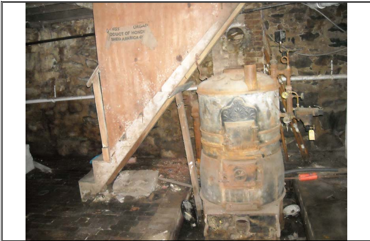
Photo 10: Old coal-burning furnace in the basement of the Site building.
