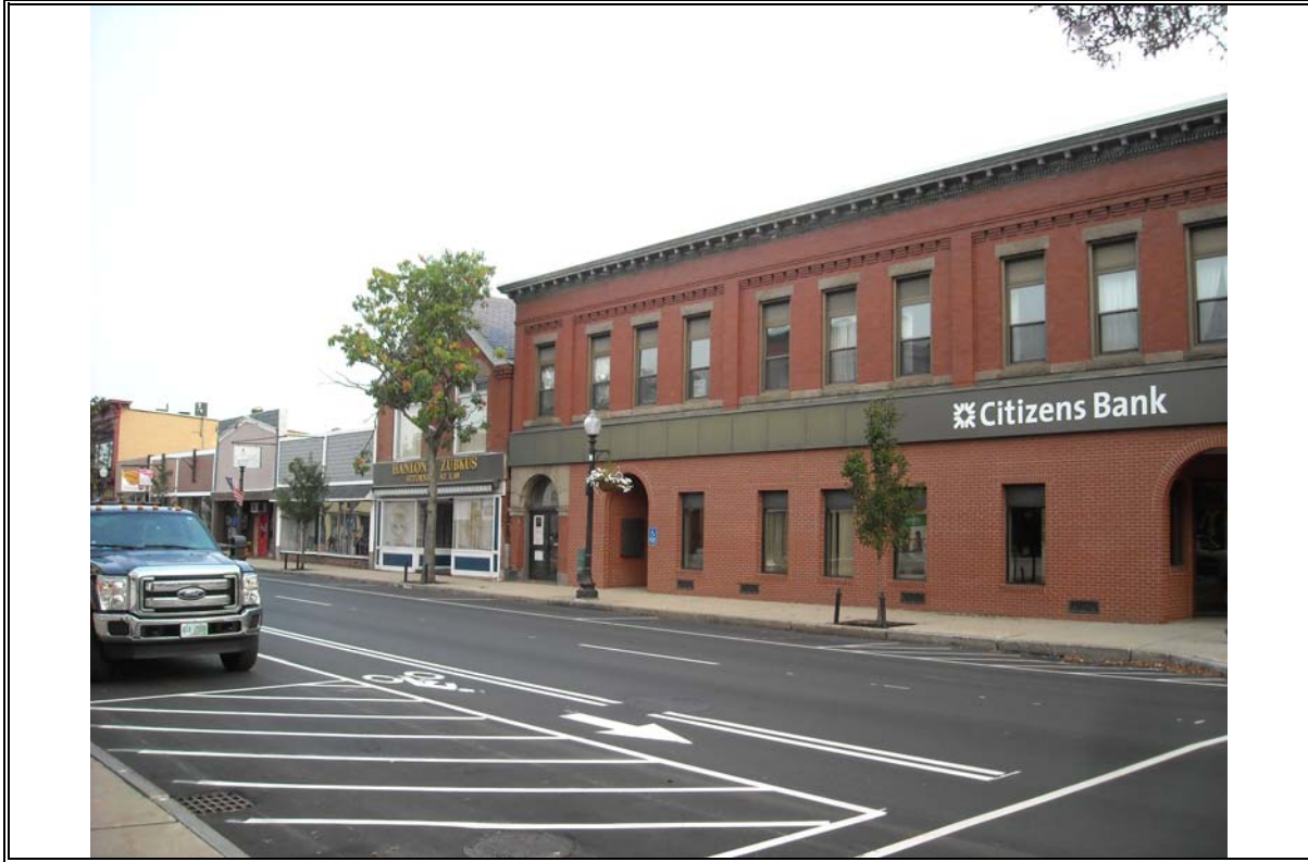
Photo 7: North-looking view across North Main Street from the front of the Site building.
