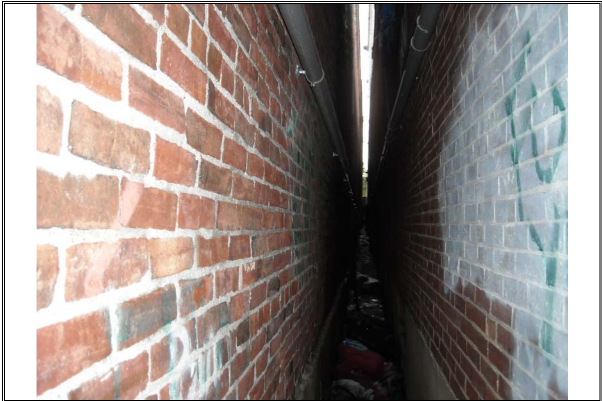
Photo 4: North looking view of the narrow space between the Site building (left) and the 10 North Main Street building (right).
