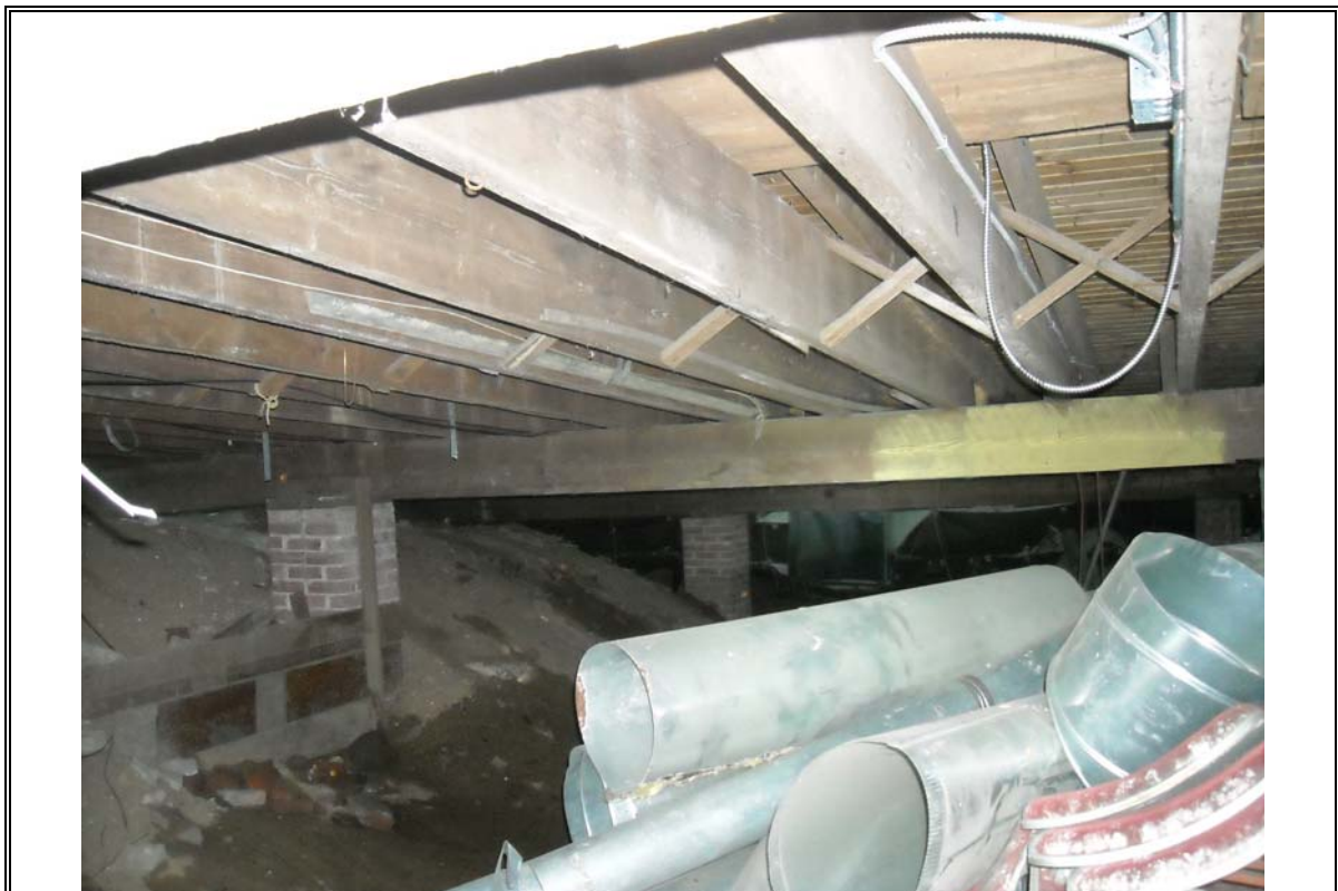
Photo 12: Discarded aluminum piping in basement of Site building.
