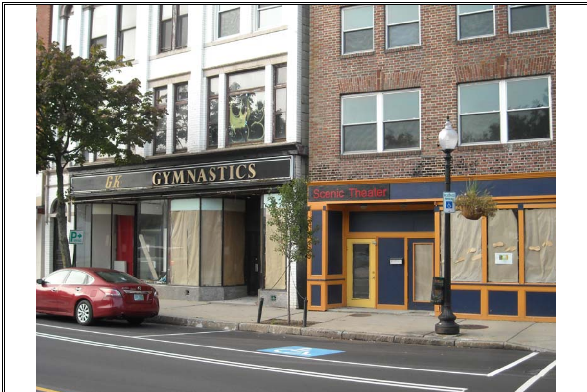
Photo 8: South-looking view of the Site building (right) and east-abutting 10 North Main Street building (left).
