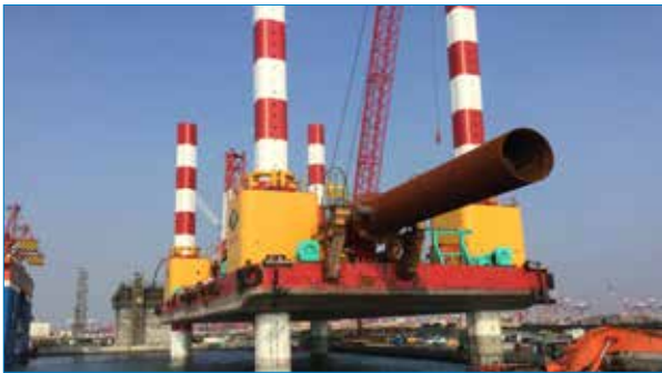
Sea Meteorological Tower under Construction
