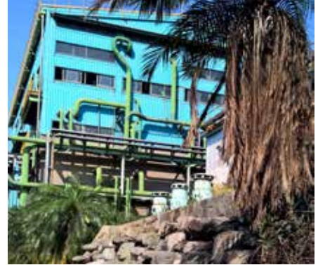
Wastewater Purification Plant
