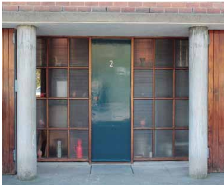
Figure 3. 1-3 Willow Road, London: The street facade. Goldfinger's house. Photograph: Catalina Mejia, © National Trust.
