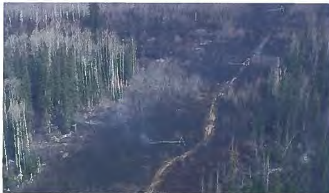
Wildfire damage to our transmission line in April 2016.
