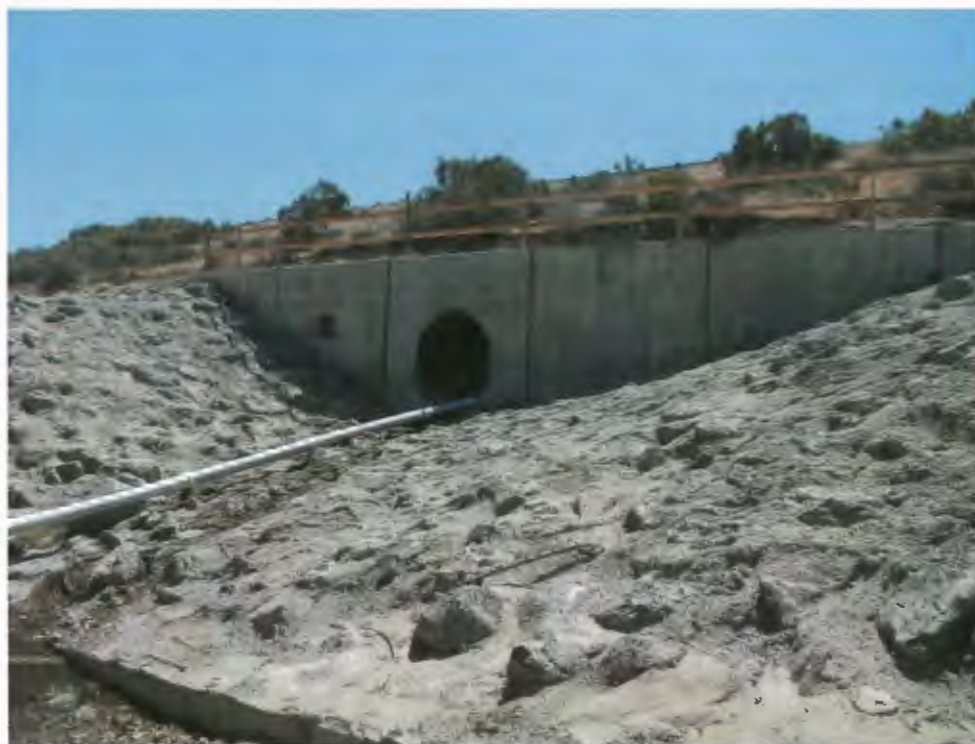
Photo 4. Feature C – Looking southeast at the culvert crossing for this feature
