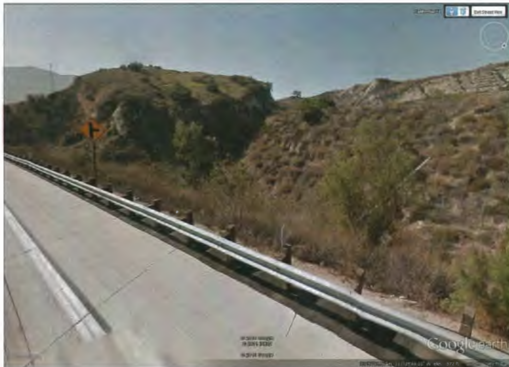
Photo 16. Feature N – Looking west at feature
