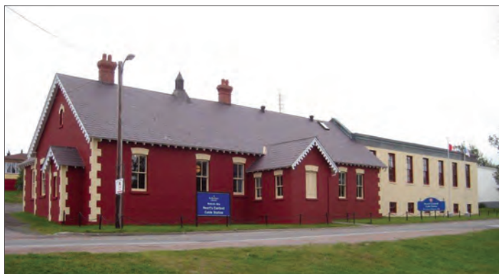
The Heart's Content Cable Station (photo by Steve Kelly, Ottawa)
