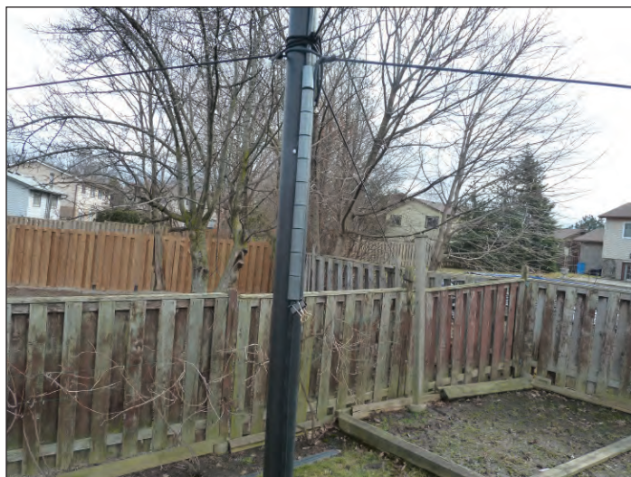
Figure 5: Ferrite Bead Balun on Feedline
