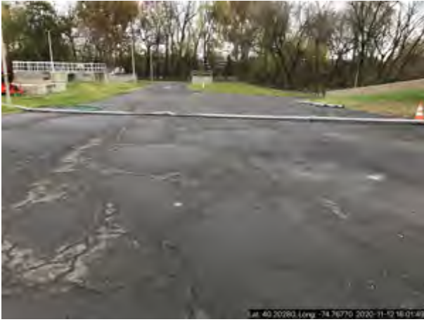
Photo #: Sludge line from DAF to Sludge Holding Tanks TP-2 3 TP Treatment Plant-0987403 A2 Description: Photo taken by BERNARD J KRASNISKY
